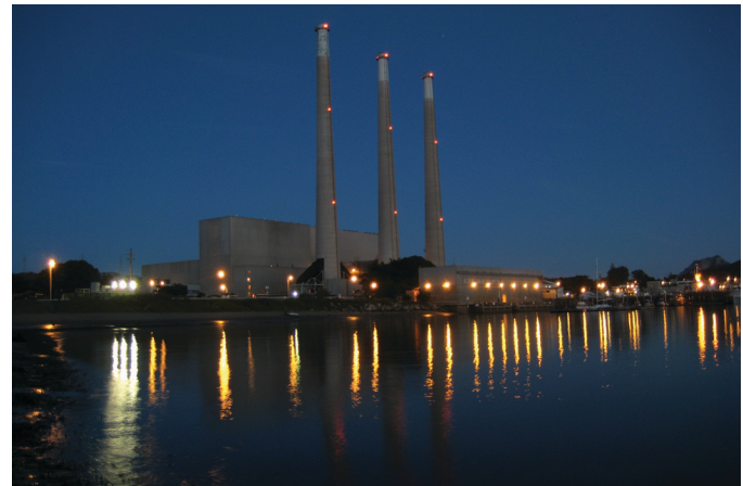
Morro Bay Power Plant © 2015 James T. Cheng All rights reserved
