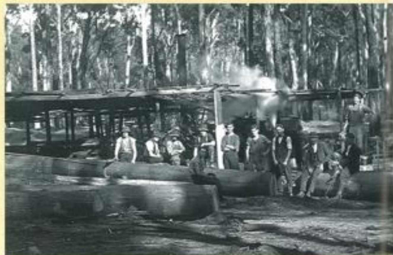
Plate 8 Oiler's Mill, near Orbost, in the 1930s. (Department of Conservation & Natural Resources collection)
