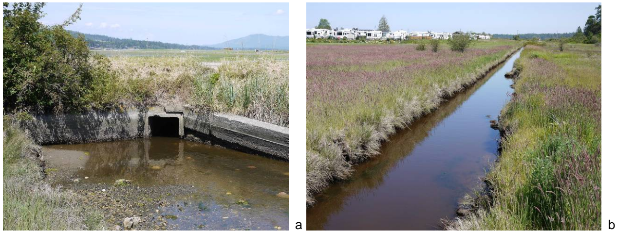
Figure 13. Examples of drainage disturbance of the Tsawout Wetland: (a) small box culvert that restricts tidal exchange into the salt marsh south of Saanichton Lagoon; (b) main drainage ditch in the north part of the Tsawout Wetland (Oceanside RV Park in background).
