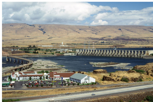
Figure 16. Dalles Dam, Columbia River near The Dalles, Oregon, 1993. Courtesy: Gary Whelan.
