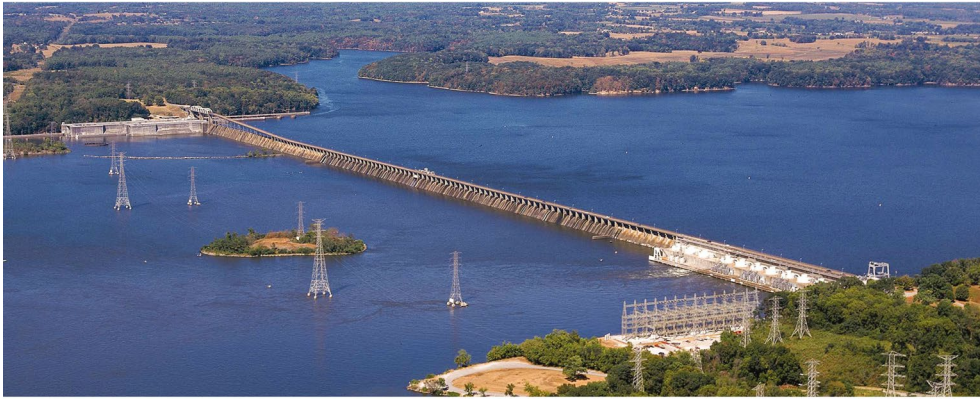
Figure 15. Wheeler Dam, Tennessee River near Rogersville, Alabama. Courtesy: Tennessee Valley Authority.
