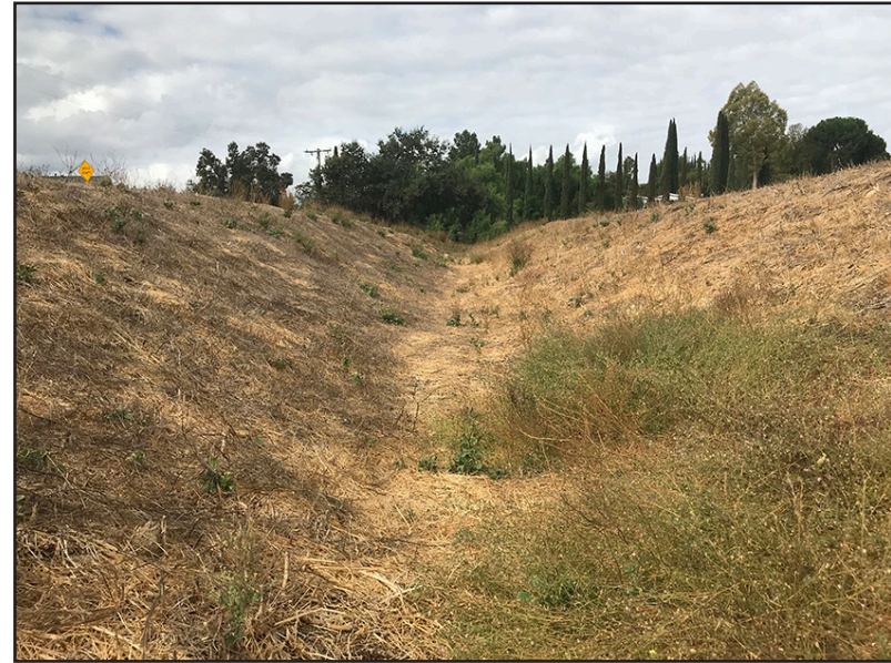
Photo 2 – View to the west illustrating Swale 2. Swale 2 is vegetated with non-native grasses and mustards. The swale terminates prior to the oak trees in the background.
