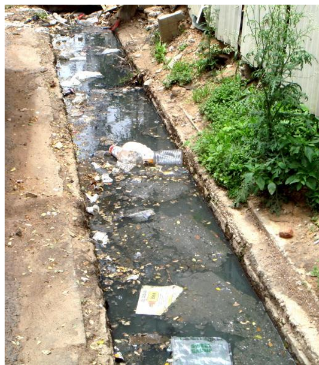
Figure 4: Stagnant water at Church Street
