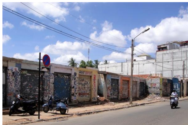
Figure 5: Raising the skyline – Low, old buildings giving way, Kamraj Road
