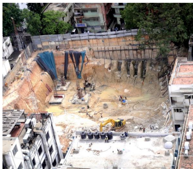
Figure 24: Construction site near M. G. Road
