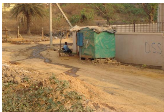
Figure 4: Disintegrating road, Peenya
