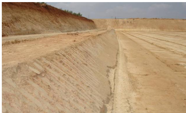
Figure 4: Landfill under construction-TSDF, Dobbaspet
