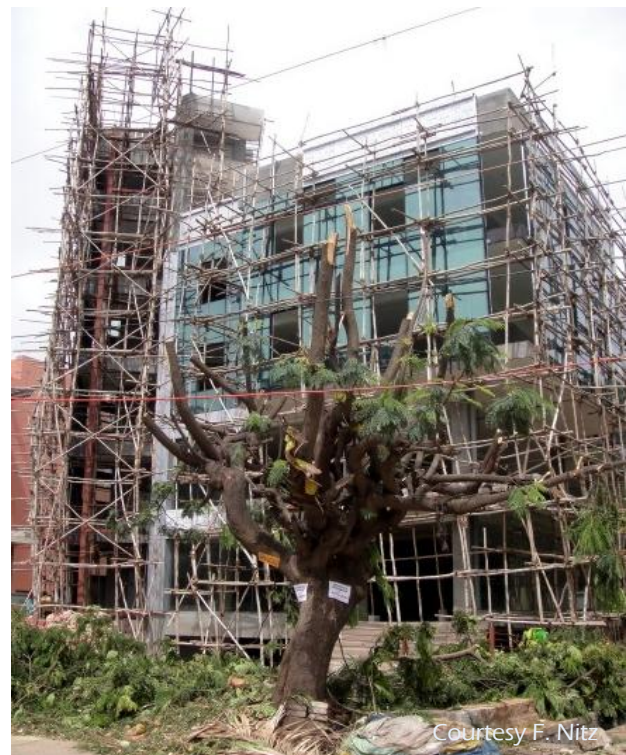
Figure 7: From branches to scaffoldings – Construction on Bannerghatta Road
