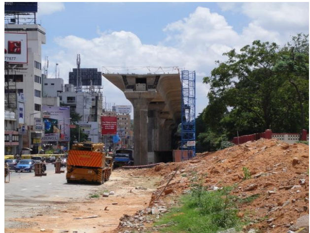
Figure 7: On the way – Metro construction at M. G. Road
