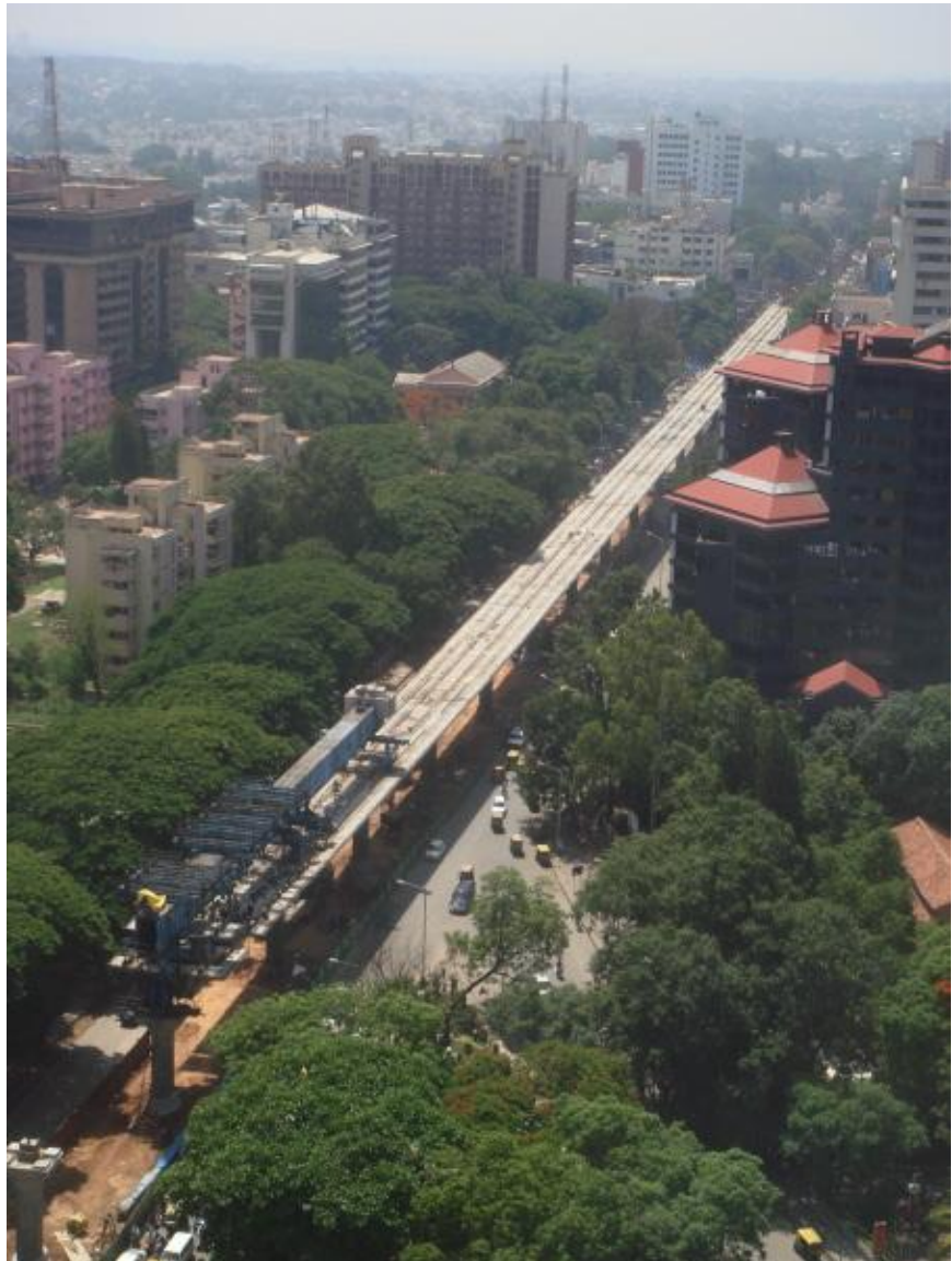
Figure 10: New horizons – Metro in the making, M. G. Road
