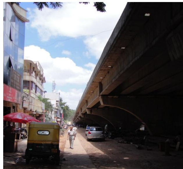
Figure 19: The up and the down side: Flyovers drastically change the perception of living space – Construction at Wheeler Road
