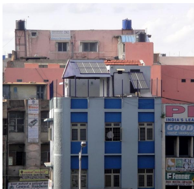
Figure 18: A rare sight – Commercial building equipped with 12 solar PV panels, generating approx. 600 W p , City Market
