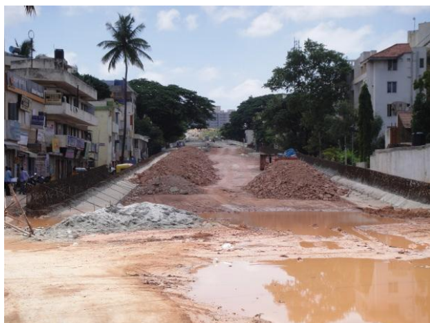
Figure 12: Fly-over in the making, Wheeler Road
