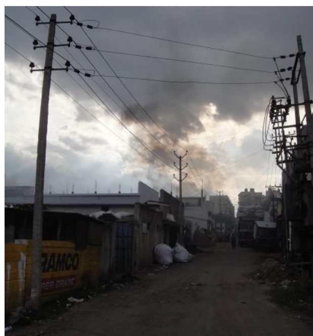
Figure 6: Private industrial area on Mysore Road
