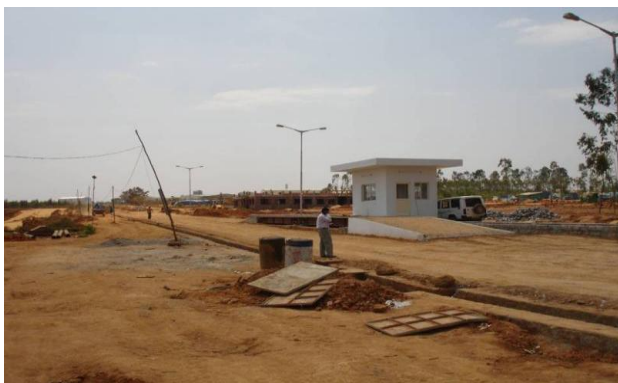
Figure 2: Weighbridge facility under construction-TSDF, Dobbaspet
