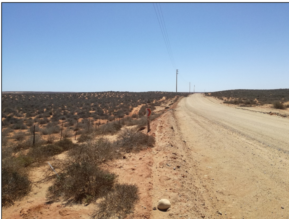
Figure B.16: View of a 66 kV power line along the Komaggas-Kleinsee link road
