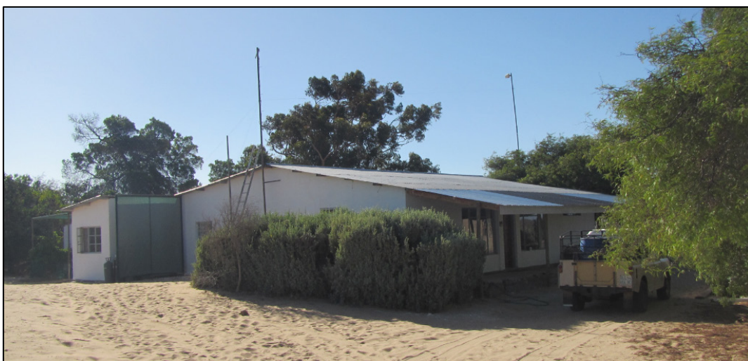
Figure B.63: Farm house on Farm 128/4 to the west of the site (photographed in 2018).
