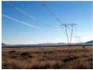
765kV Transmission Pylon @ 1000m
