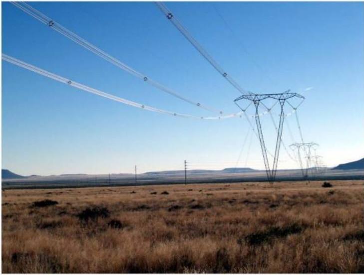
765kV Transmission Pylon @ 250m
