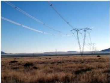
765kV Transmission Pylon @ 500m
