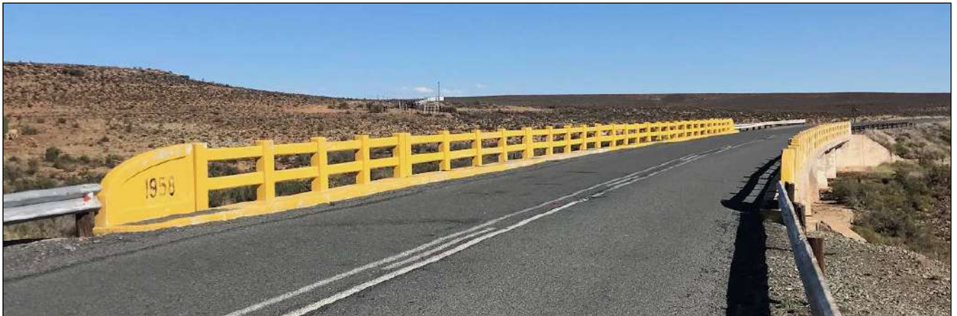
Figure 6.5 BTC07 - Bridge over the Soutpoot River (1958)
