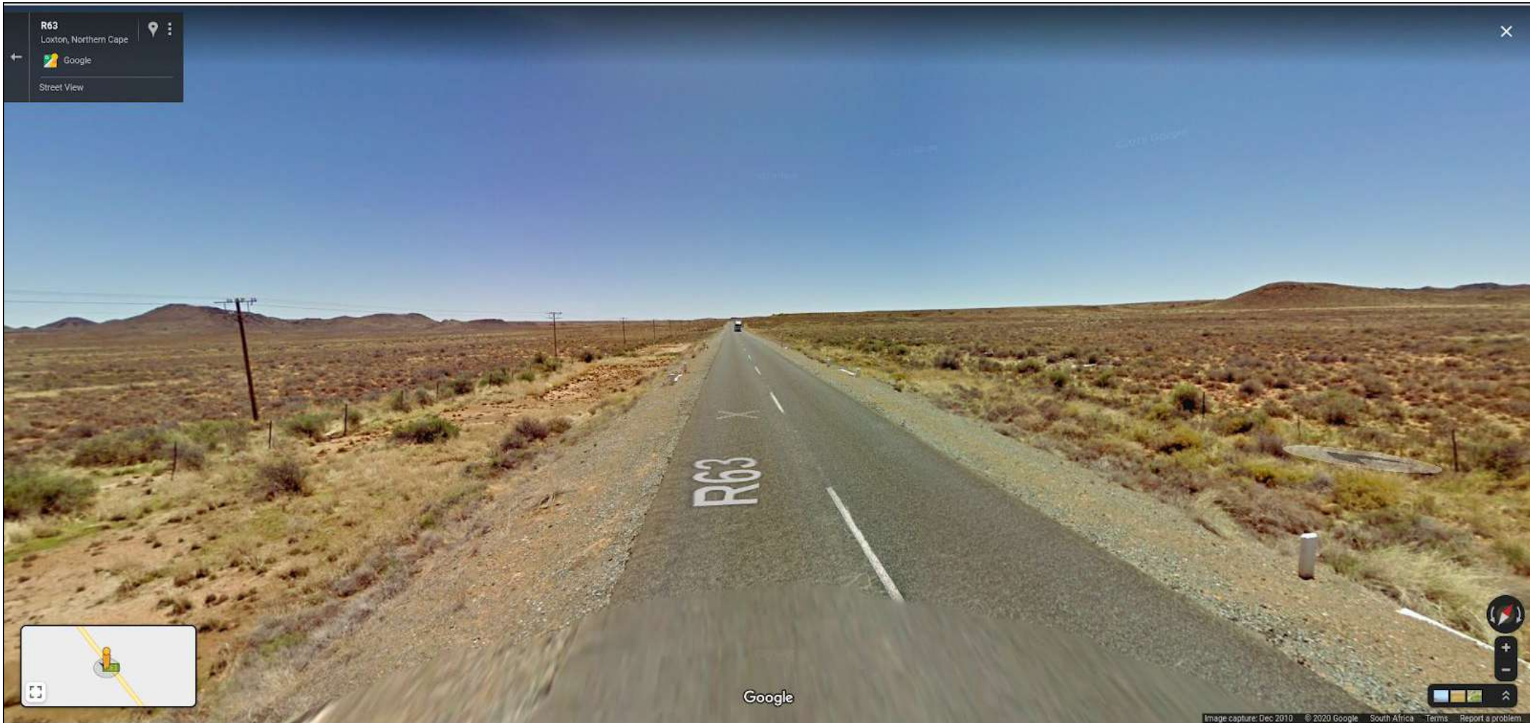
Figure 6.3. Contextual Images. Facing north along the R63 - Google Street View
