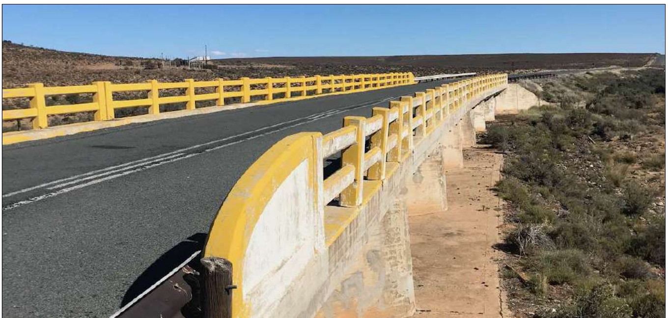
Figure 6.6 BTC07 - Bridge over the Soutpoot River (1958), northern side with basic structure evident
