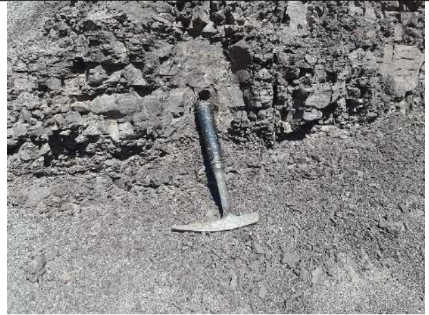
Figure 19 Highly fractured mudstones
