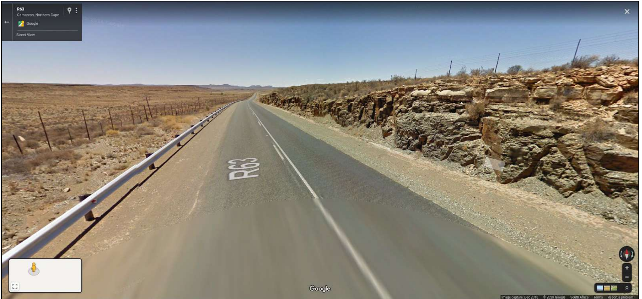
Figure 6.5 Contextual Images. Facing north towards Carnarvon along the R63 - Google Street View
