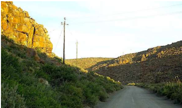
The 22kV Eskom powerline crosses the R381 Route twice over a short distance in the scenic Blounek Pass
