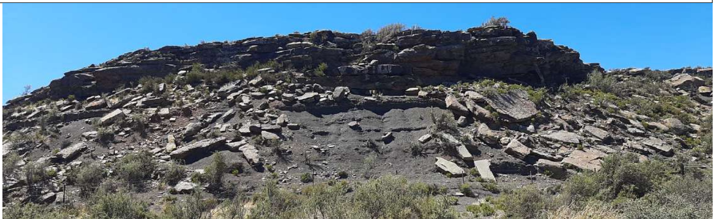
Figure 15 Road cutting showing highly fractured mudstones, with more resistant sandstone, note how the broken sandstone sheets cover much of the finely fractured mudstones
