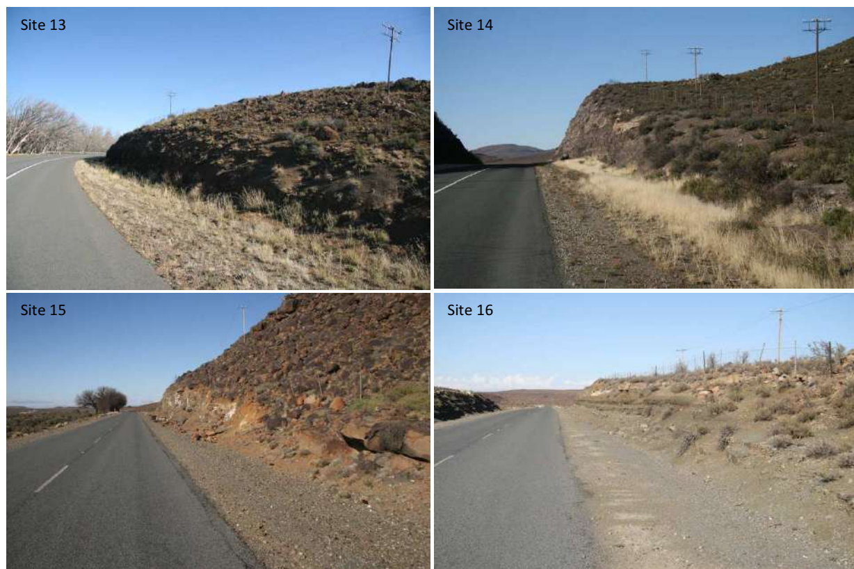
Figure 41: Instances on the underground section where trench where the trench cannot go over the cutting, but should be next to the road. (a) Site 13; (b) Site 14; (c) Site 15; and (d) Site 16 (see text for GPS co-ordinates).
