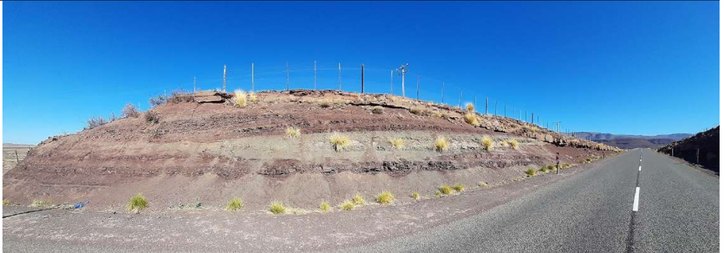
Figure 13 Road cutting showing highly fractured mudstones, with more resistant sandstone
