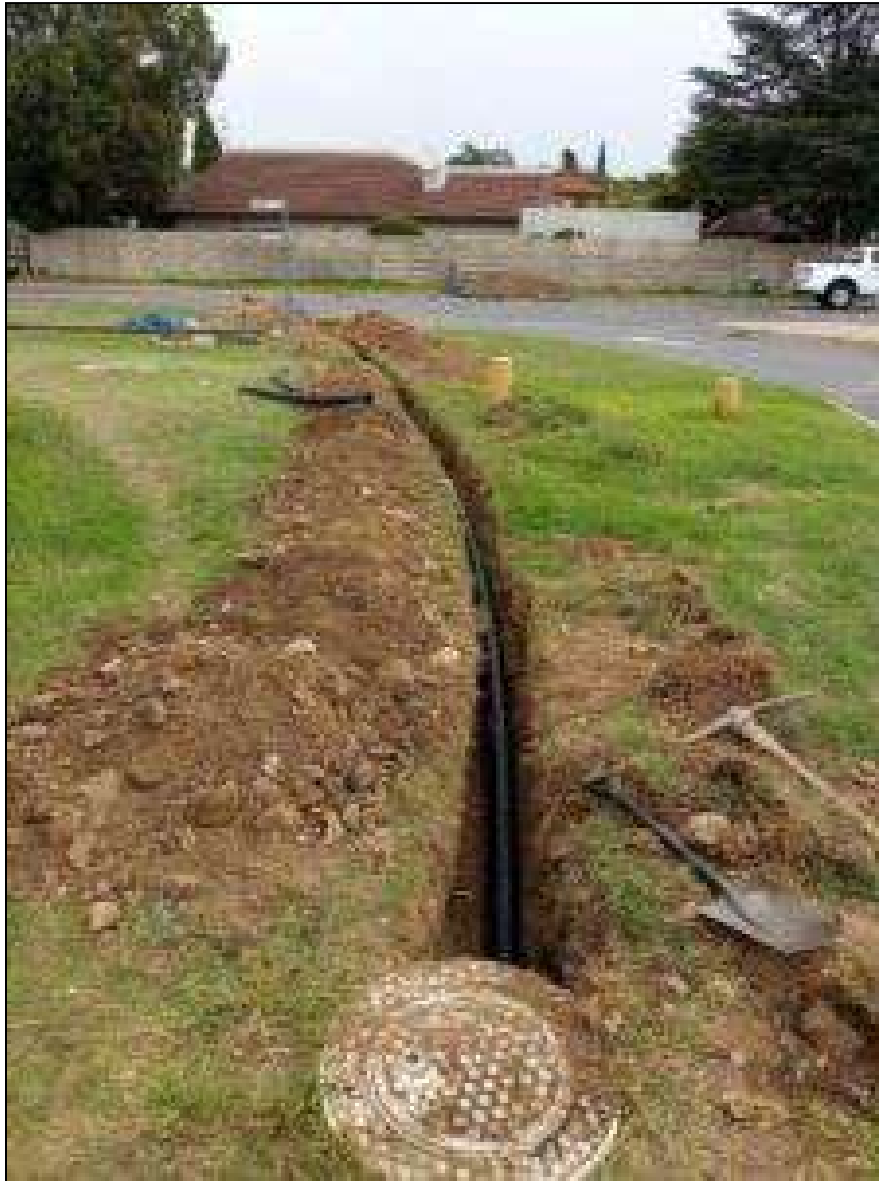
Figure 7.1 and 7.2 Infrastructure. Photos showing typical underground and overhead fibre optic cable installation
