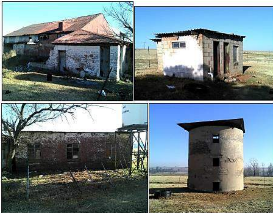
Figures 9 to 12: Buildings to the south of the R50 road. Only the large shed at upper left seems to have been present in 1945.
