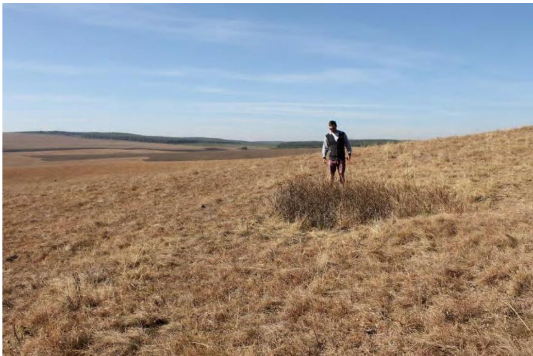
Figure 13. Piping, which serves to recharge wetland environments, present on site
