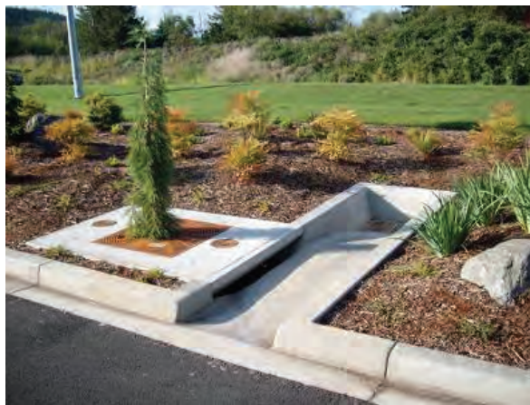
Figure 10 - Examples of Constructed Tree Boxes
