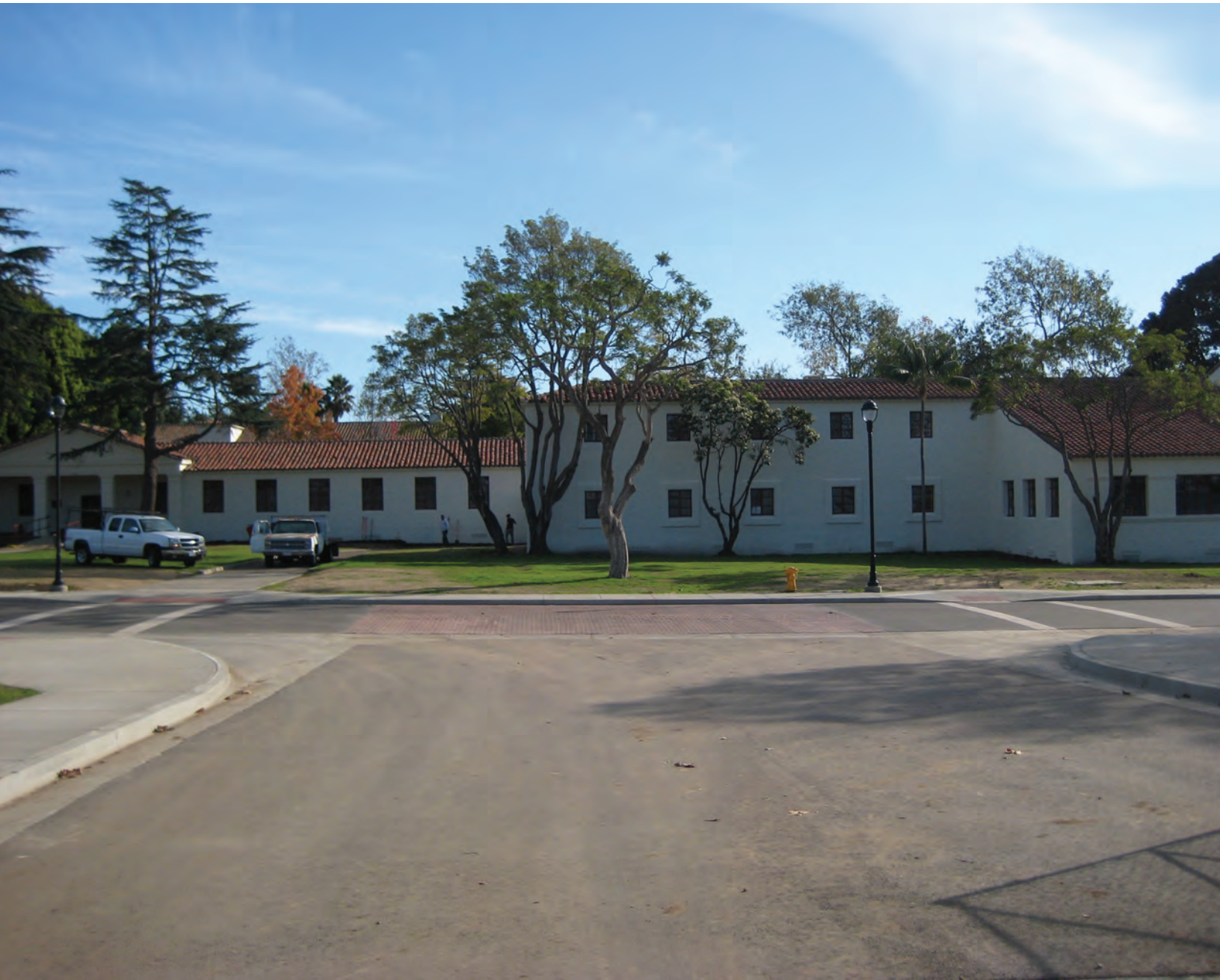
Existing view from University Drive where it meets Santa Barbara Avenue
