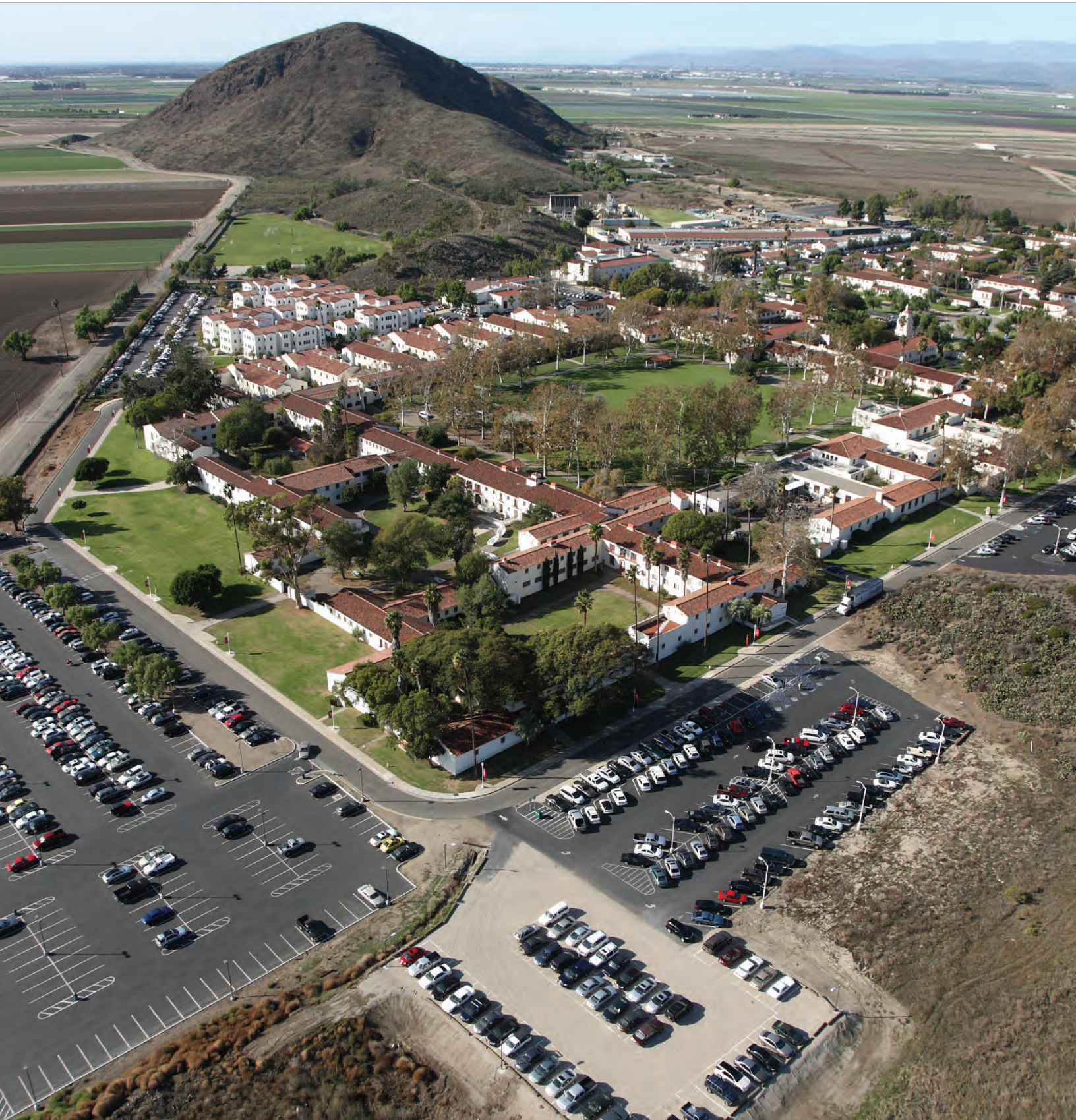
Existing view looking west
