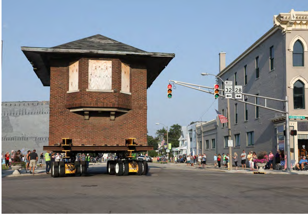
The former CSXT Interlocking Tower in Union City, Indiana, makes its way toward its new home in a city park. (Zach Marlow)
