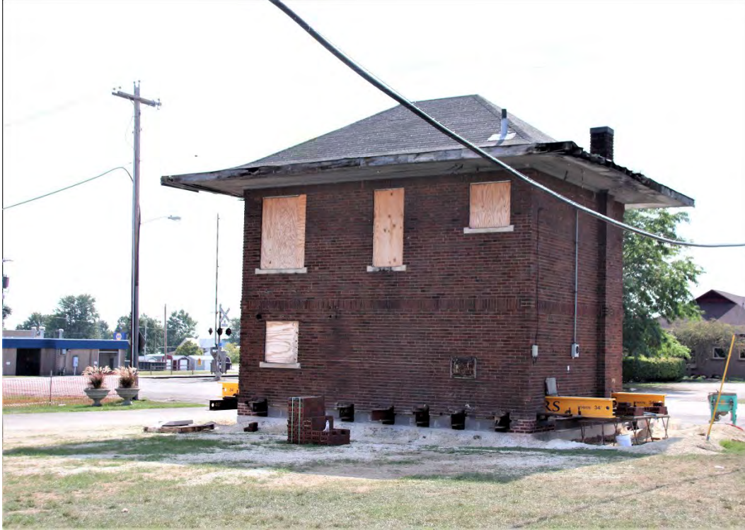
The Union City Interlocking Tower in Artisan Crossing Park. On the left is the CSXT track. On the right can be seen the former Pennsylvania Depot now a local art center and museum.
