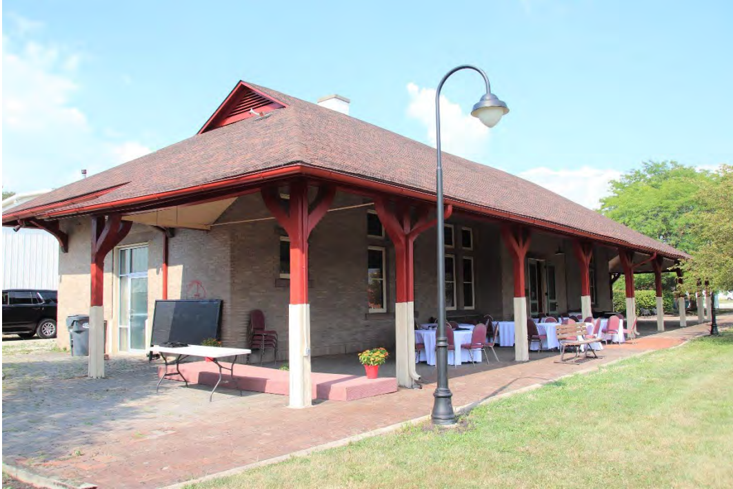
The remodeled Pennsylvania Railroad Depot that now serves as the community arts center.
