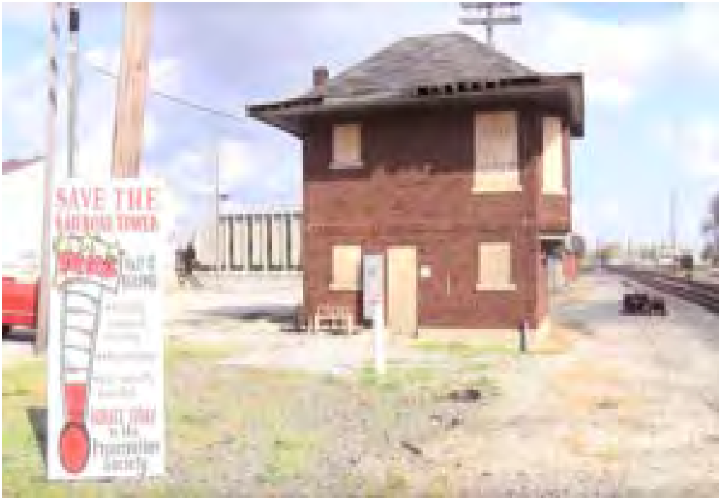
The tower sits trackside in early 2021 with a thermometer recording the amount of money donated to save it. (Union City Visitor Center)
