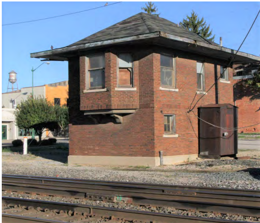
View of the Union City Interlocking Tower before being moved. (Steve Salamon)
