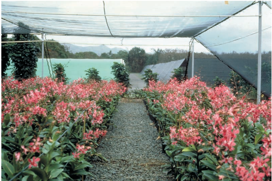
1.2. A typical pipe-and-cable shadehouse structure with diagonal side curtains. The diagonal cable connects the top of each perimeter pole to an anchor.
