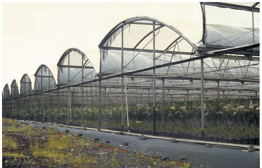
1.1. Plastic-covered structures with open sides for maximum ventilation allow best management of moisture in the nursery environment. Modern aluminum-frame structures are durable and relatively inexpensive.
