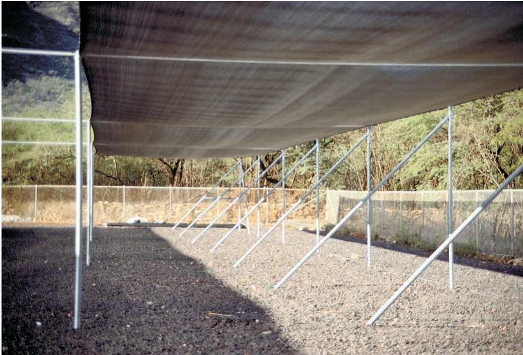
1.3. Pipe-and-cable shadehouse structure with vertical sides. Interior diagonal steel braces replace the cable-to-anchor design of structures with diagonal side curtains. Vertical sides allow better use of nursery floor space at the perimeter, but the structure is more prone to wind damage.
