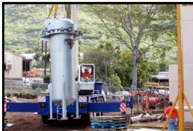
Figure 34. Flash carbonization unit located on the UH campus.
