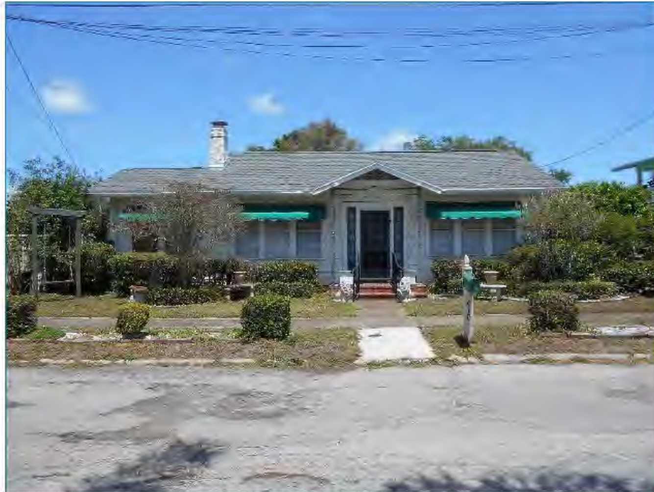
Figure 65: Minimal Traditional house at 410 W Lemon Street.
