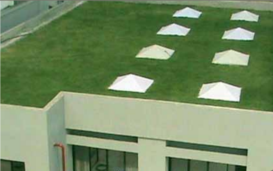
Landscaping on the canteen roof of the Ranjangaon facility.
