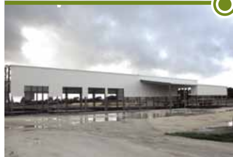
Mount Gambier, Australia (under construction)
