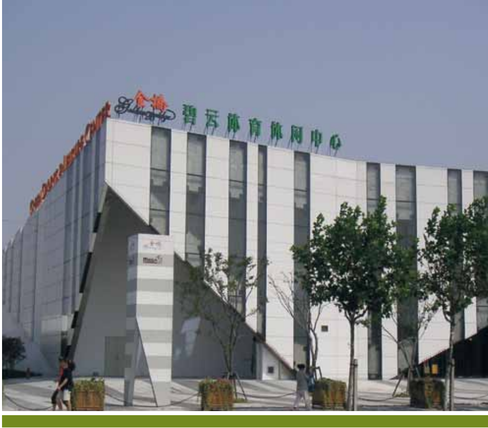
Cummins Power Generation's combined heat and power cogeneration system powers the Jinqiao Sports Center, a 120,000 square foot sports facility in Shanghai, China.
