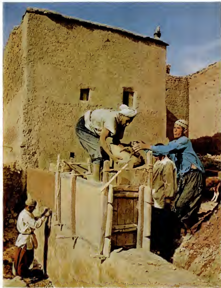
BUILDING A HOUSE , Berber tribesmen dump mud into a wooden mold. The mud is pounded down until the mold is full. The sides are then removed
