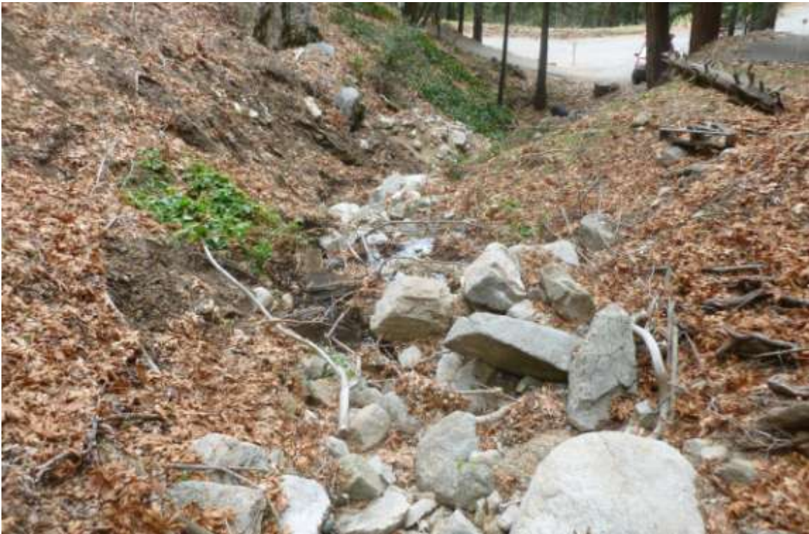
Photo 2. General condition of site. View facing west-southwest.
