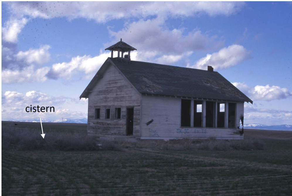
Figure 22. Highland School. Cistern in foreground. Source: Author photo, March 1998.
