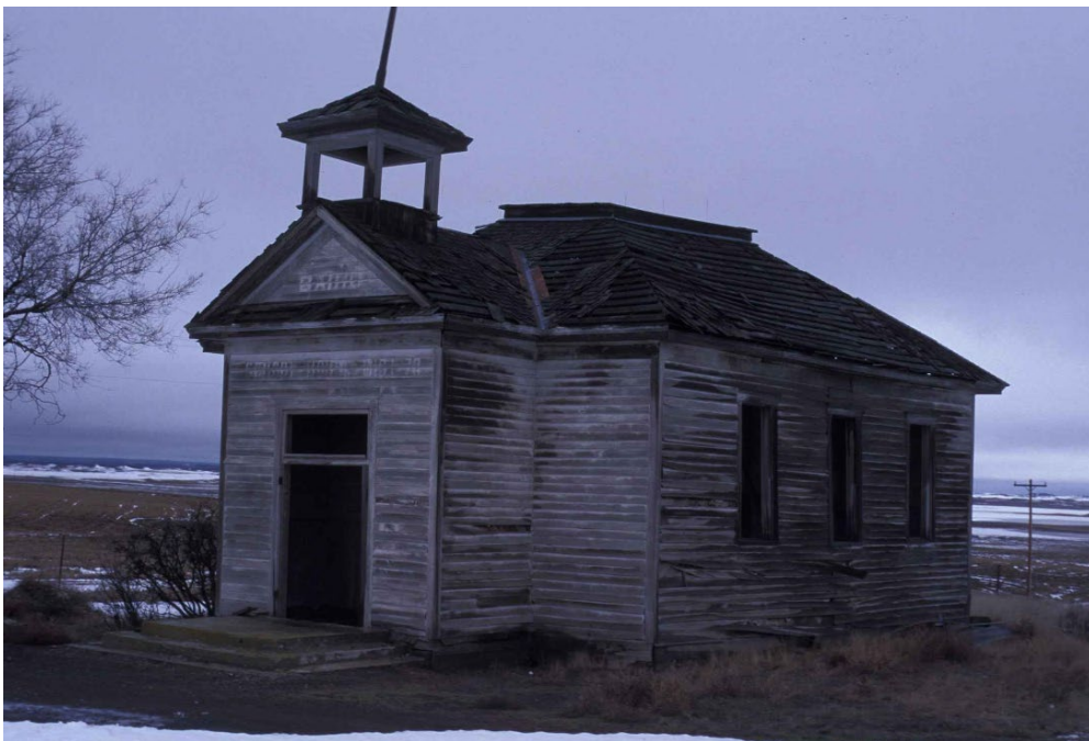
Figure 23. Baird School as of March 2000, view northeast. This structure apparently dates back to before 1915 when it was located 1.75 miles east. Source: Author photo.
