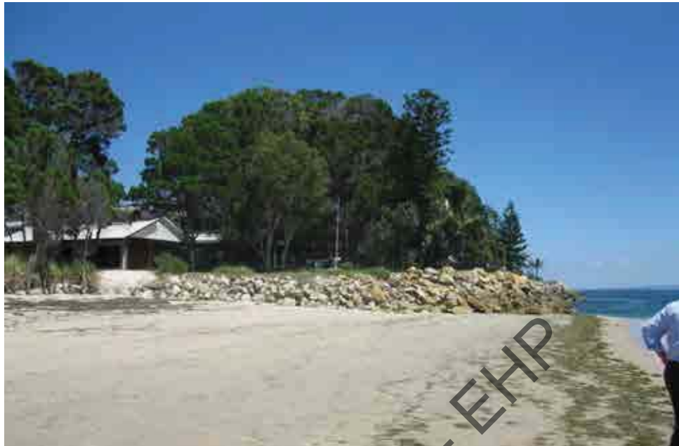
Figure 5-1 Rock Revetment near Amity Point (Source: NearMap Pty Ltd, 2011)
