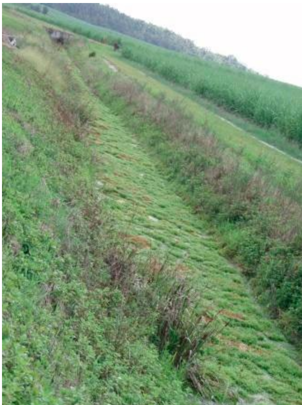
Figure 11. Table drain blocked by Mayaca fluviatilis alongside sugarcane near Innisfail (photo: Audrey Reilly and Kylie Goodall, DERM).
