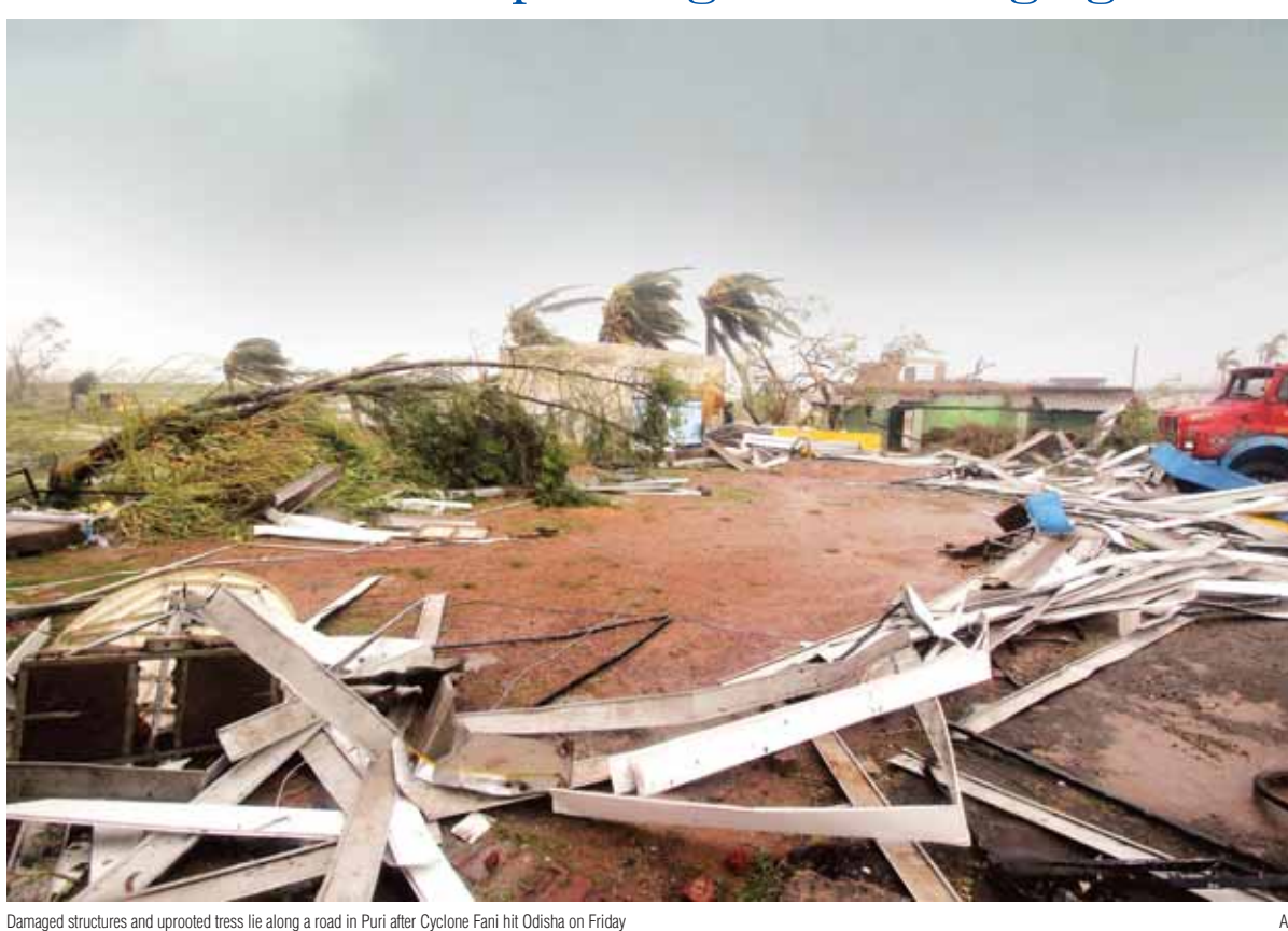
Damaged structures and uprooted trees lie along a road in Puri after Cyclone Fani hit Odisha on Friday
