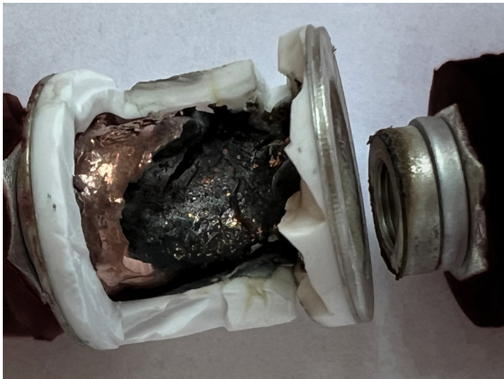
Figure 9c. Internals of failed spark gap tested at 3700Arms. The sample failed shorted.
