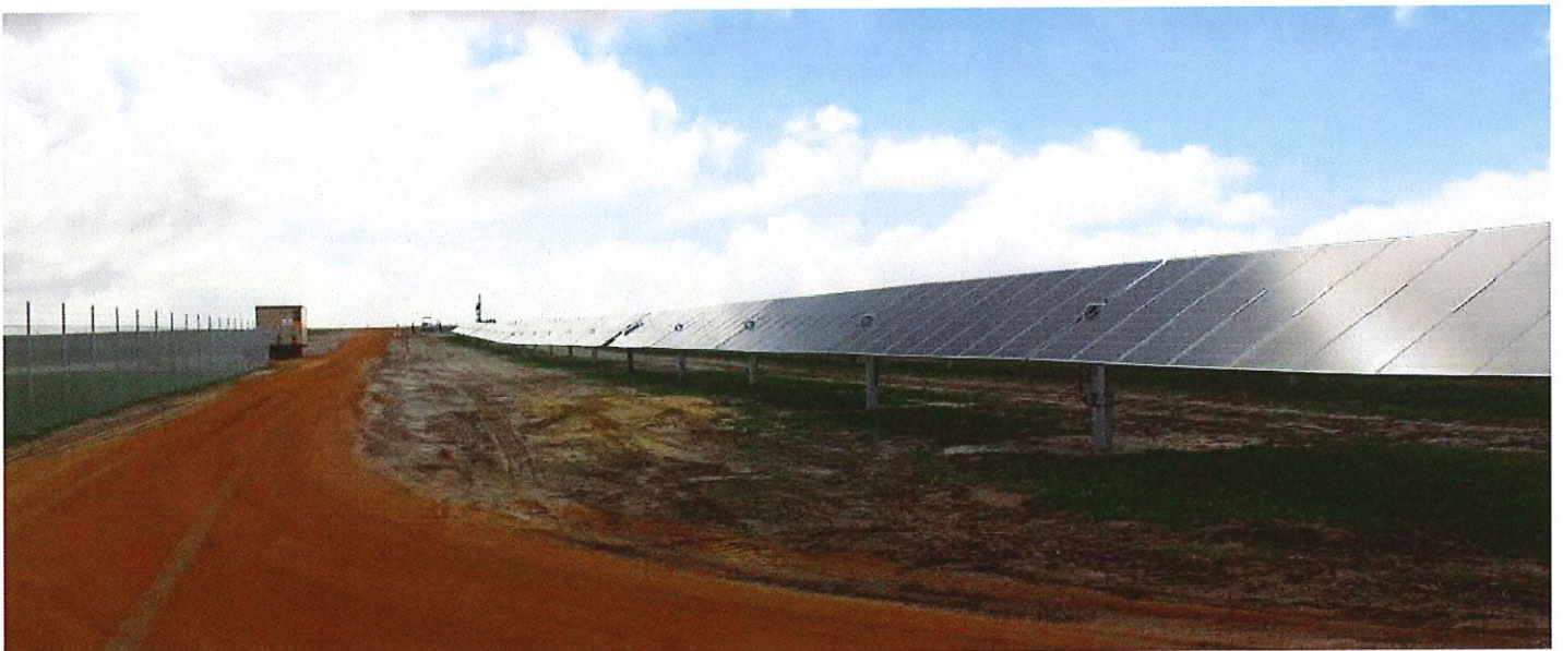
Emu Downs Solar Farm
