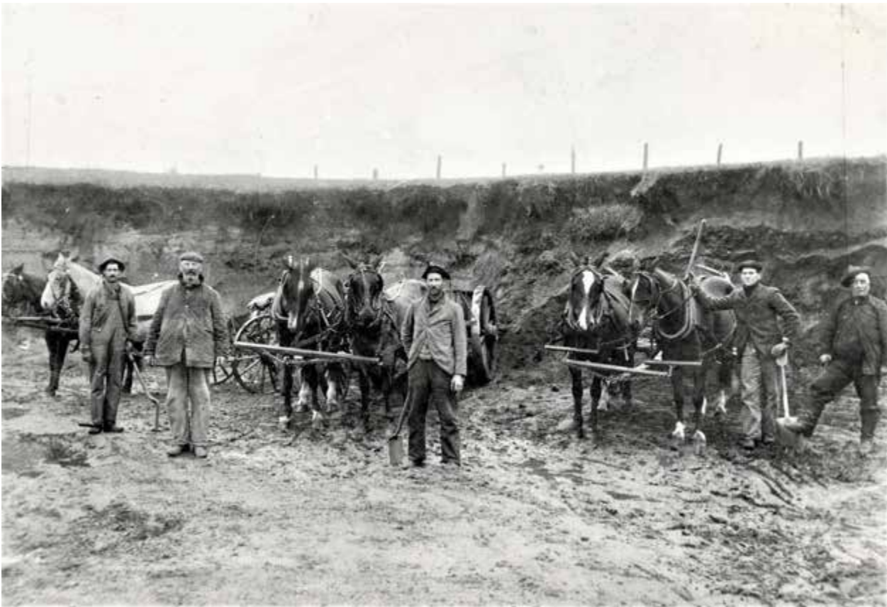
The Danville gravel pit was located on the former site of Joe Peck's duck pond, on the right side of Route 2 heading toward West Danville, in the early 1900s. Town workers stand at the ready with their shovels as their teams of horses patiently wait to draw the wagonloads of dirt to their destination. The crew are from left to right: Fred H. McCosco, Noel Burdick, Henry Weeks, Bert Heath, Bert Hartshorn. Danville Historical Society
