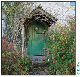
Fig 5 : Beneath the entrance canopy at Church House is an arched granite 16th century door frame.
