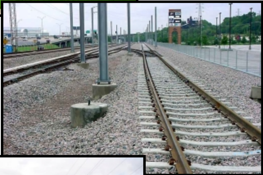
Trackwork in Northern Part of Project
