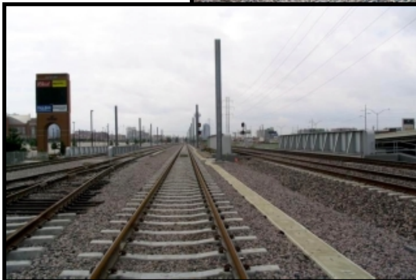
Hi Line Bridge
