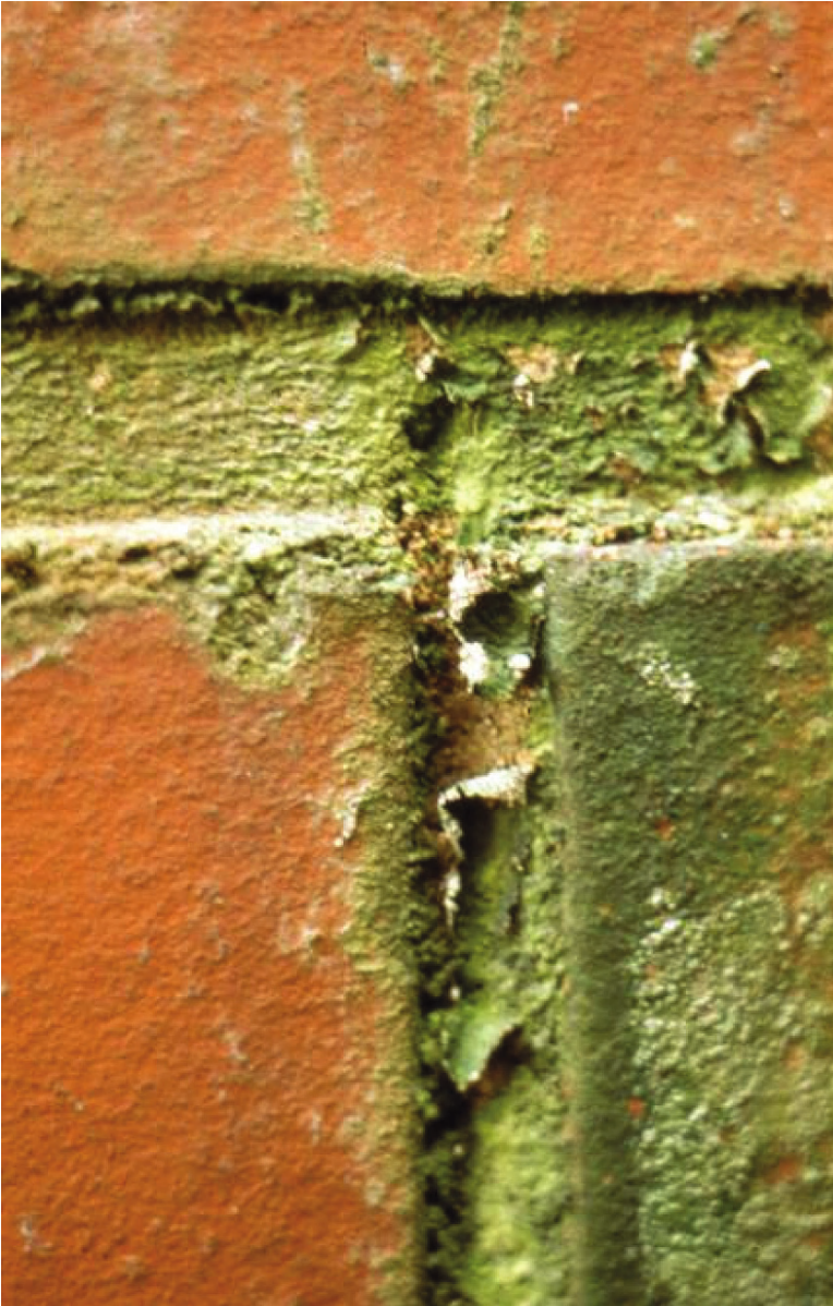
Fig. 3 Desiccated biofilm. The cohesive forces and the surface adhesion forces increase. Curling of biofilms occurs and sand grains from mortar are ripped out, contributing to microbially influenced weathering
