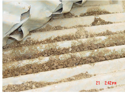
b Dry Deposits on Fills
