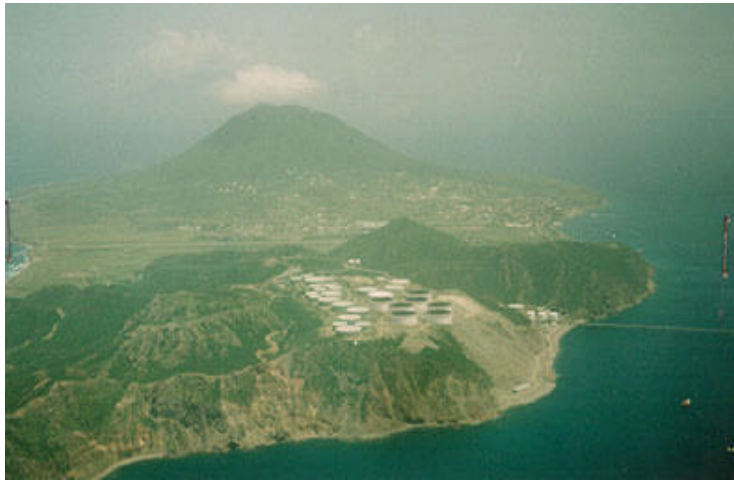
Photo 4. Aerial photograph of the Oil Terminal and Tumble Down Dick Bay.
