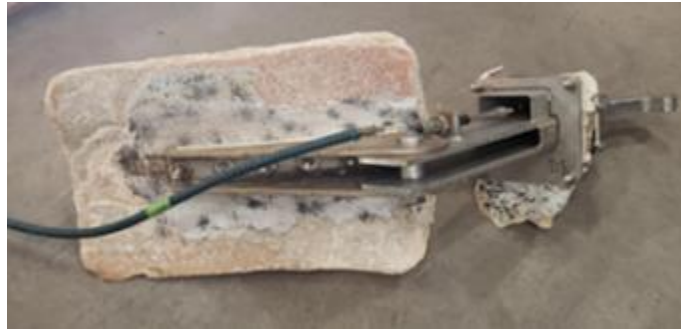
Figure 21: Bow hook and surrounding FRP post-casualty. Credit: CG.
