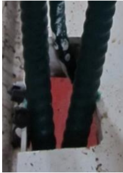
Figures 38 (left) and 39 (right): Photos of aft control cables in or around 2014. Credit: Shell.
