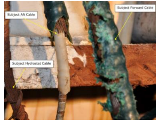
Image 7: Photograph of aft control cable after casualty. Photograph documents separation of three layers of the conduit: the green plastic cover; a steel wire; and a white polyethylene liner. Credit: DNV-GL.
