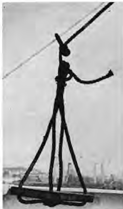
FAULTY METHOD of rigging bosun's chair suspected of contributing to fatality.
