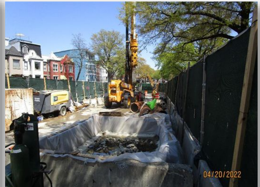
Junction Manhole Construction
