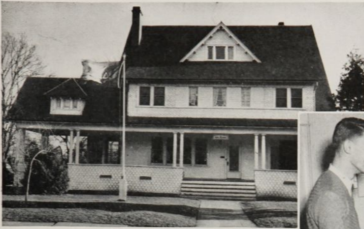
Delta Shelter at 716 Boyer Avenue, Walla Walla, Washington.
