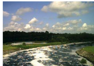
S. Florida Water Management District 147 MOBOTIX Kameras, USA
