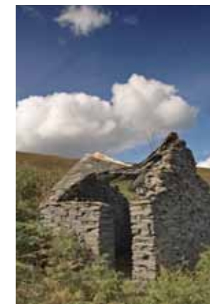
Hen adeilad chwarel An old quarry building
