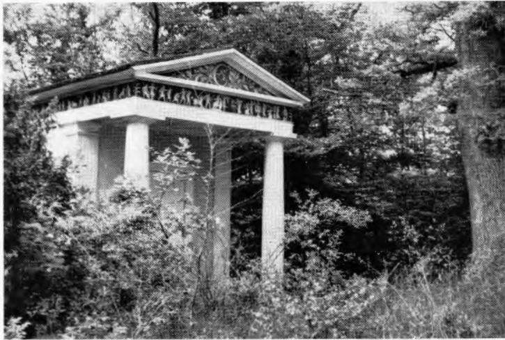
Fig. 3. Skärva. "Grönastugan". — Foto N.-Å. Ekeroot. — Skärva. The small pavilion called "the green cottage" in neoclassic style from about 1790.
