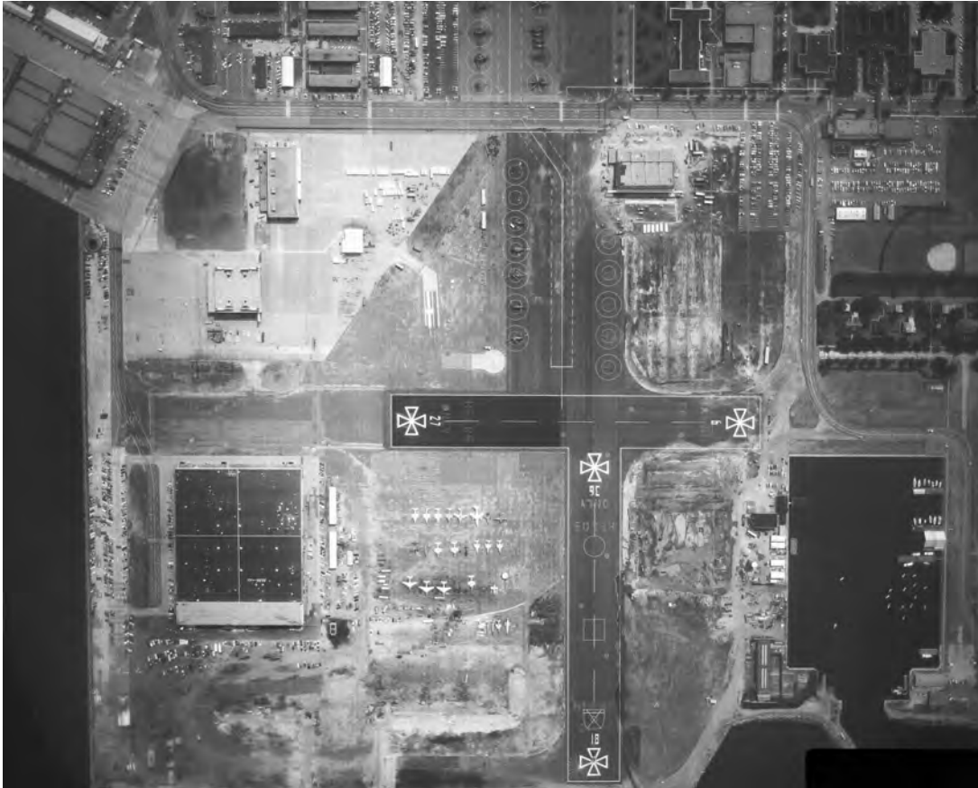
FIGURE 4-10. AN AERIAL VIEW OF THE OLD HELICOPTER PORT AT NORFOLK NAS, JANUARY 1, 1979
