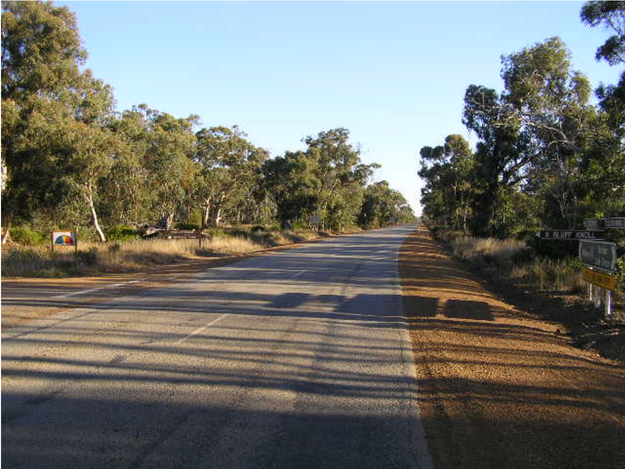
PLATE 1 - View south along Albany – Lake Grace Rd from intersection of Bluff Knoll Rd
