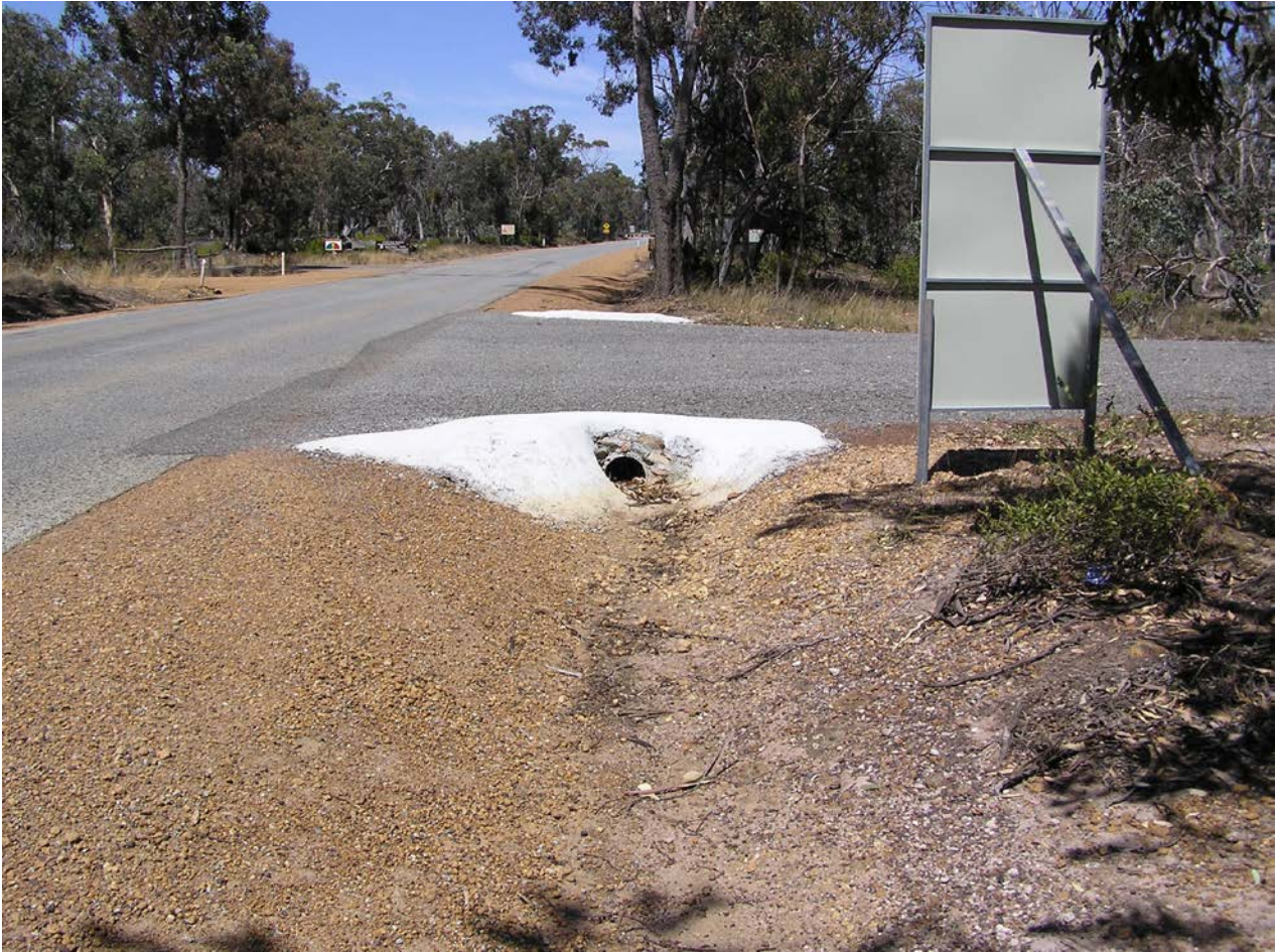
PLATE 4 - View to south along Albany – Lake Grace Rd looking towards Bluff Knoll Rd intersection showing existing driveway on western side of Albany – Lake Grace Rd and vegetation on verge which will need to be cleared to allow for construction of the proposed auxiliary right turn lane.
