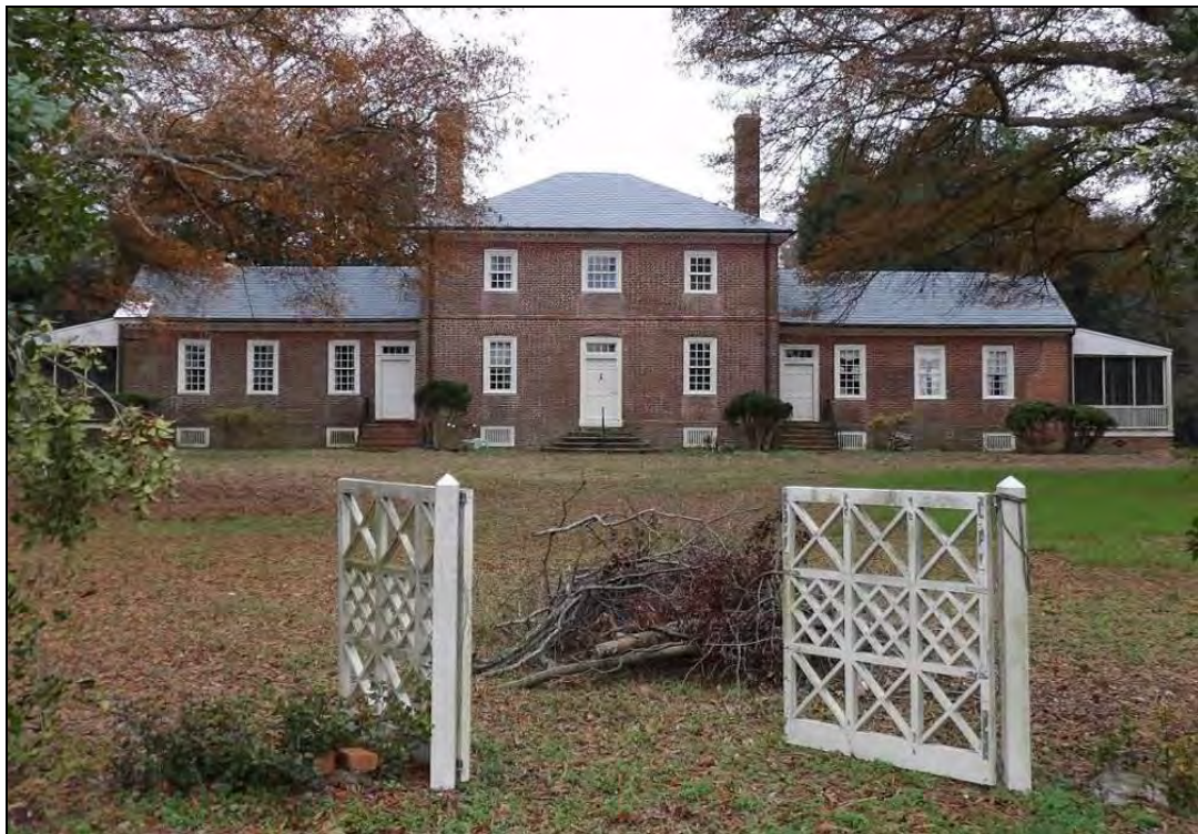
Photo 1: Northeast Elevation of the Belle Isle Mansion at Belle Isle State Park (051-0001).
