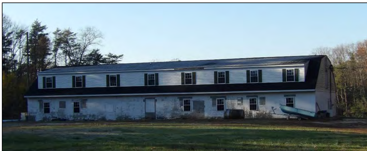
Photo 14: Northeast Elevation of Fish or Oyster Processing Warehouse at 497 Doggett Lane (051-5250).
