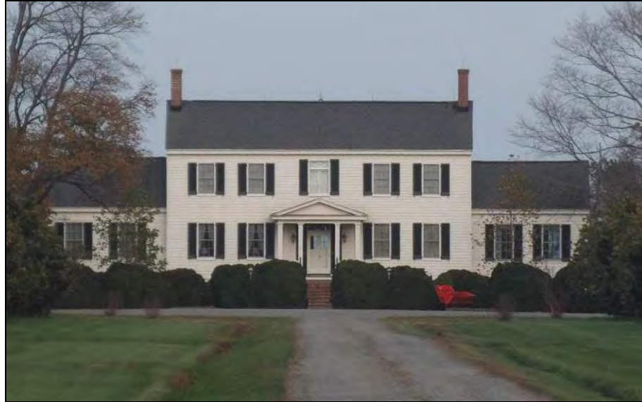
Photo 19: West Elevation of Gascony (066-5054).
