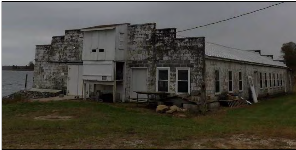
Photo 26: Northwest Oblique of an Oyster Processing Warehouse on Mila Road (066-5112).
