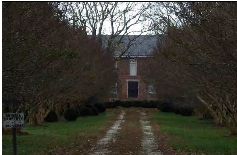
Photo 16: West Elevation of Cobbs Hall (066-0003).
