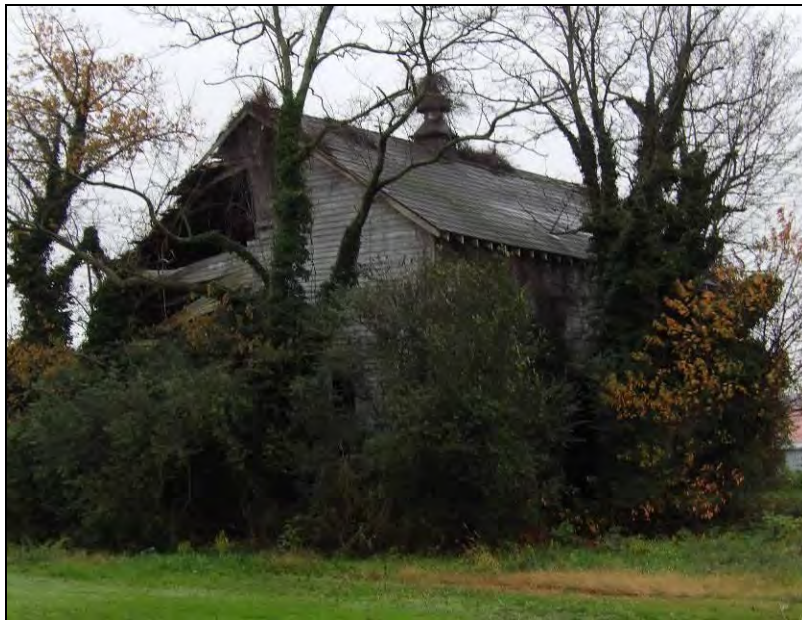
Photo 25: West Oblique of Abandoned Barn on Wicomico Point Road (066-5097).
