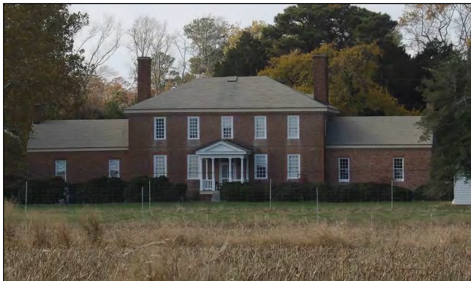
Photo 17: East Elevation of the House at Ditchley Plantation (066-0004).
