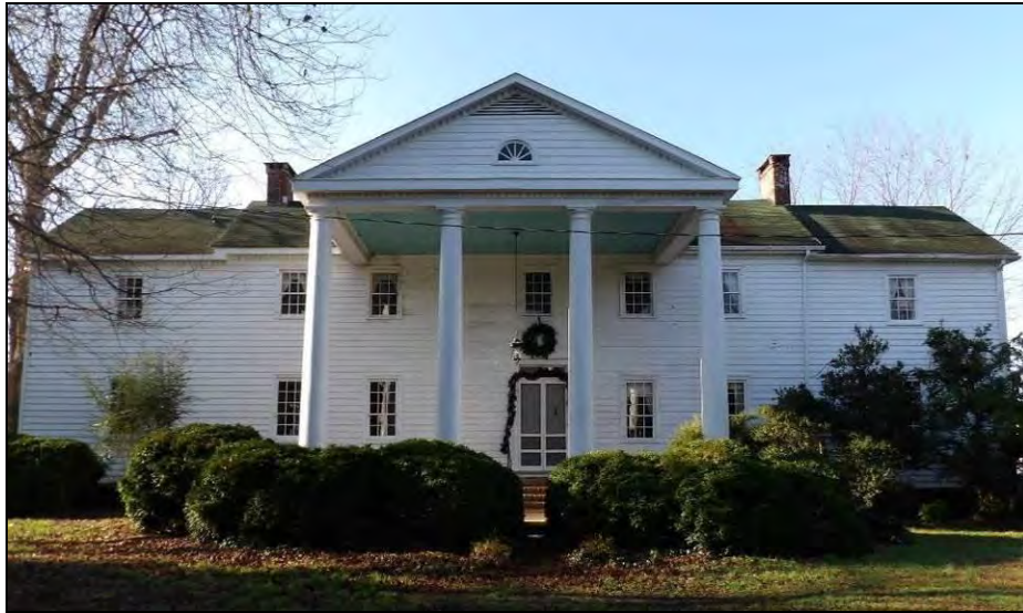
Photo 7: Northeast Elevation of the Locust Grove House (051-0124).
