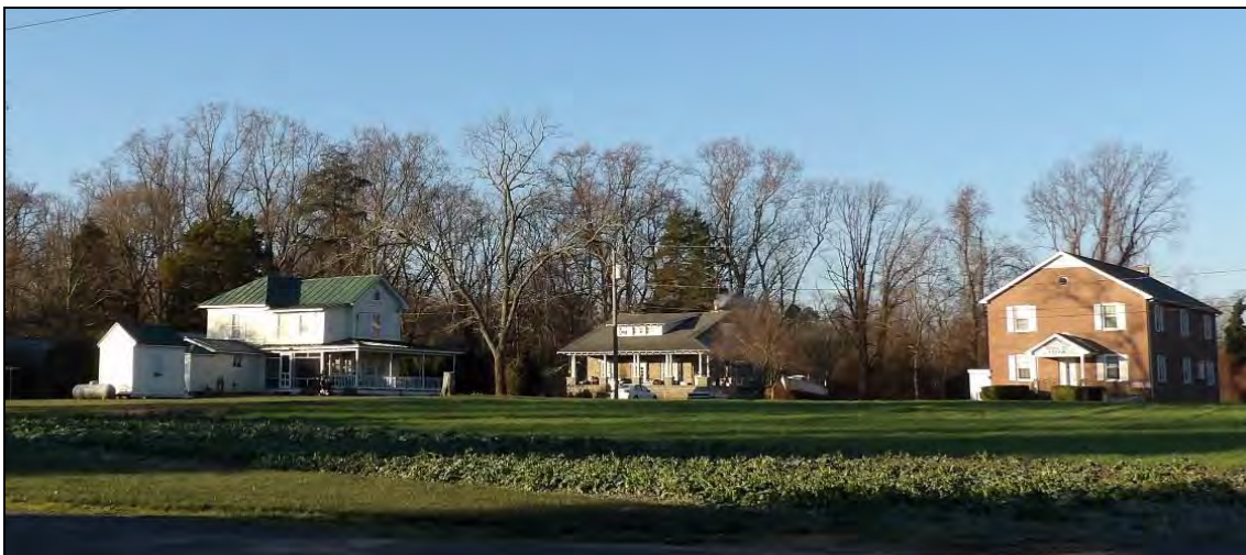
Photo 27: South Side of Great House Road in Kinsale Historic District (096-0090).
