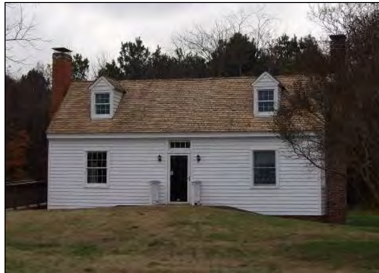
Photo 6: Southwest Elevation of the Belle Isle Park Office (051-5092).
