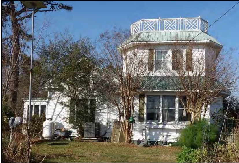
Photo 9: Southeast Elevation of the House at 232 Oyster Creek Drive (051-5228-0003).
