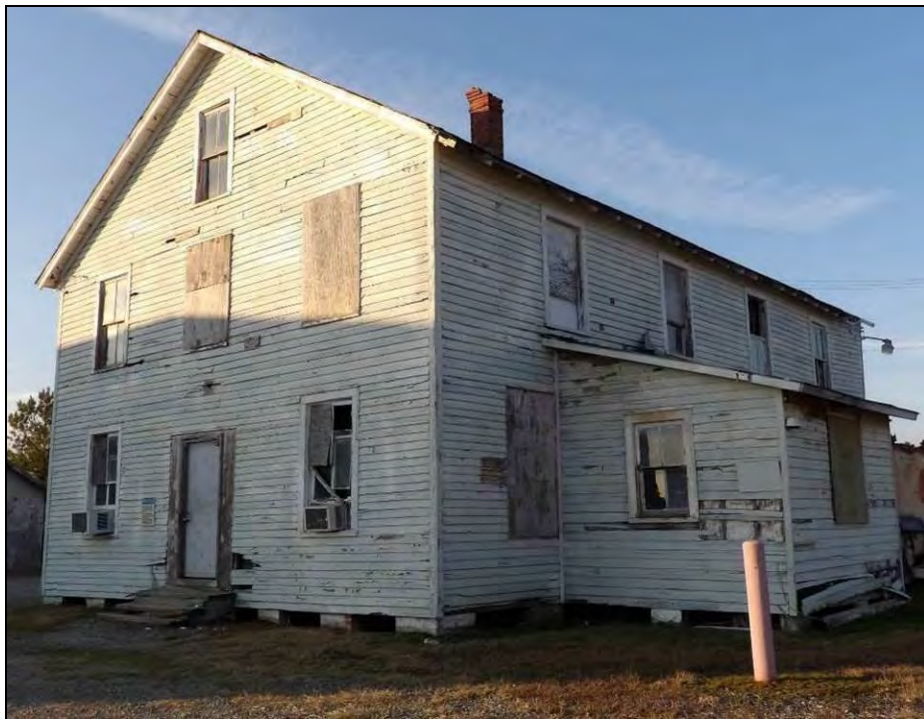
Photo 8: Northwest Oblique of Office Building at AMPRO Shipyard Company (051-0212).
