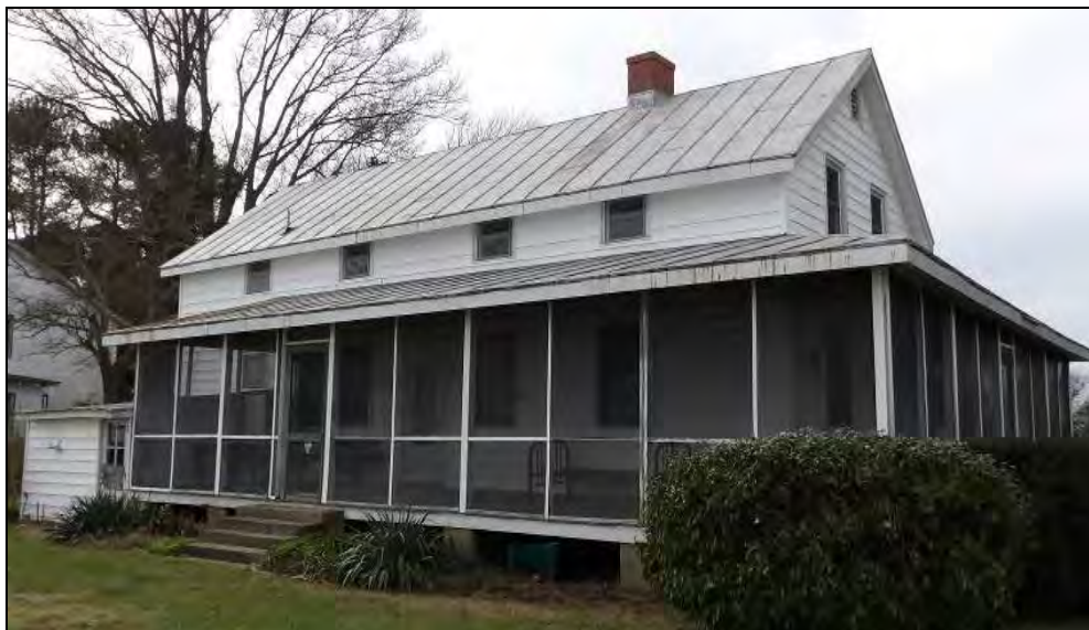
Photo 38: Example of a Circa-1920 Waterfront Cottage, Hartshore Cottage (096-5204), North Oblique.
