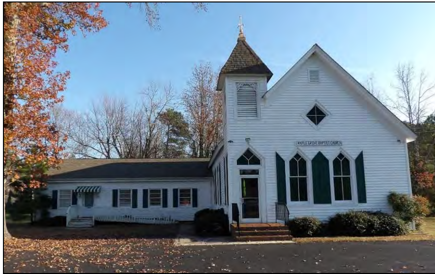
Photo 15: Northwest Elevation of the Maple Grove Baptist Church (051-0156).
