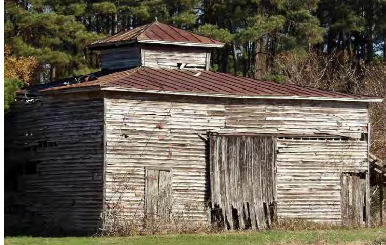
Photo 5: Southwest Oblique of the Barn at Chownings Ferry Farm (051-0003).
