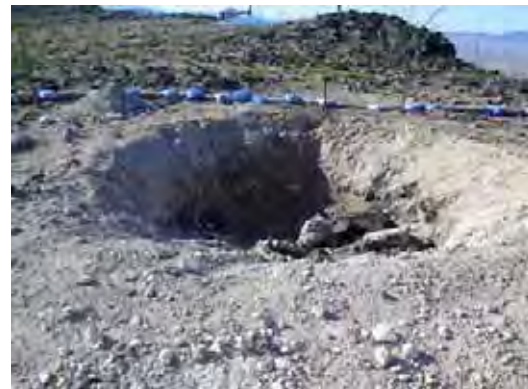
Photograph 1-2. Excavated hole at TCA-AJO-189
