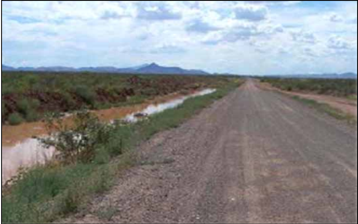
Figure C-3. FC-2 All-Weather Road (Photograph)
