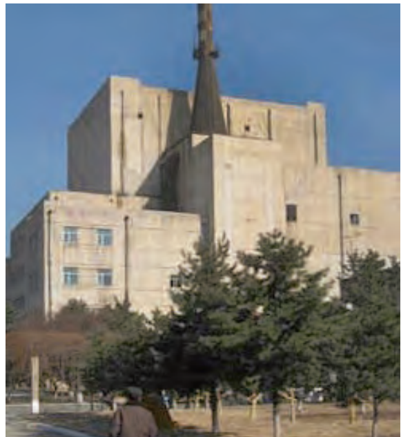
Reactor at the Yongbyon Nuclear Research Complex. North Korea has acknowledged both plutonium reprocessing and uranium enrichment activities at this installation. Activities at Yongbyon sites continue.
