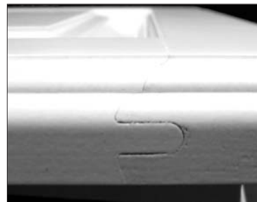
Example of end joint separation
