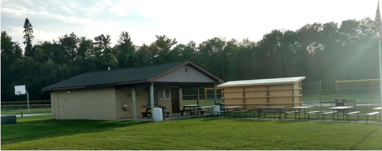
Existing Ballfield Complex (new dugout under construction)
