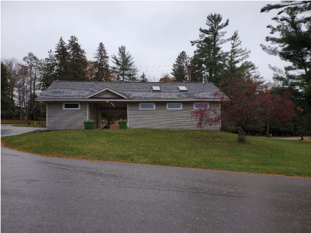
New shower/restroom building
