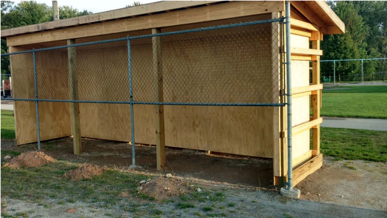
New Dugout under construction
