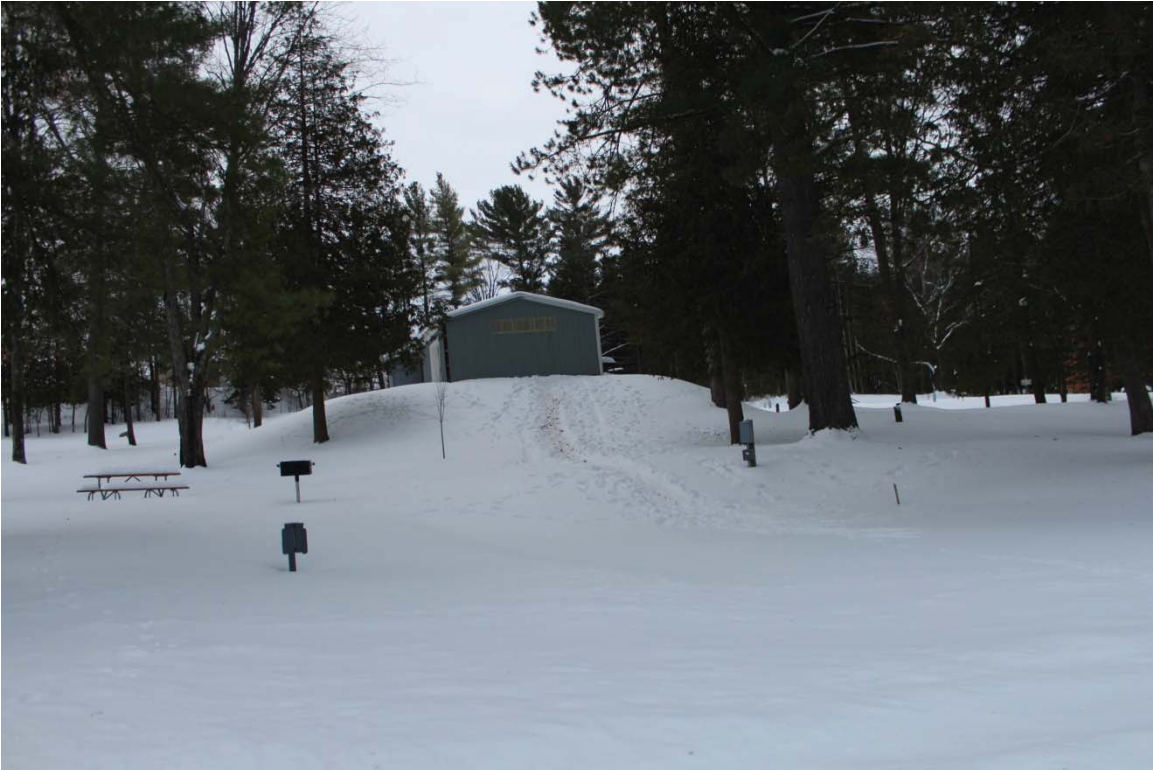
Original restroom/shower building now converted to maintenance garage
