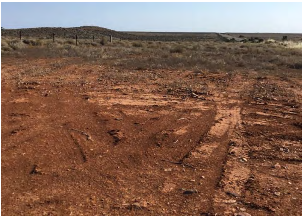
Figure 10 Minor rutting at proposed site access point
