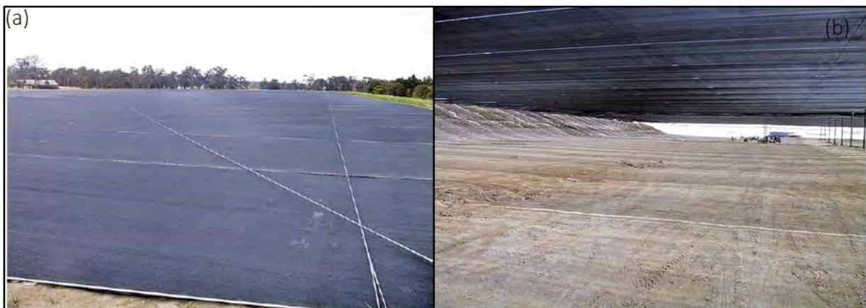
Figure 9: Example of a static evaporation cover viewed from (a) above and (b) below.
