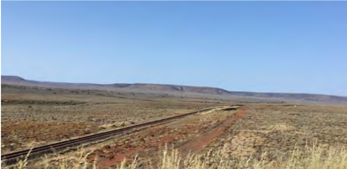
Figure 13 Existing access track adjacent rail (and proposed water supply pipeline)
