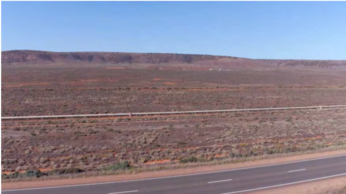
Figure 5.6 SA Water Storage facility (drone images)
