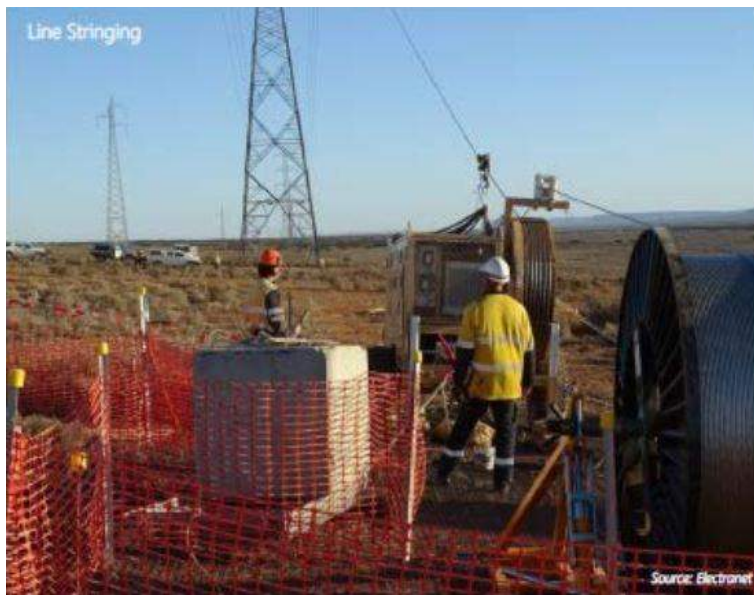
Figure 4: Typical line stringing equipment
