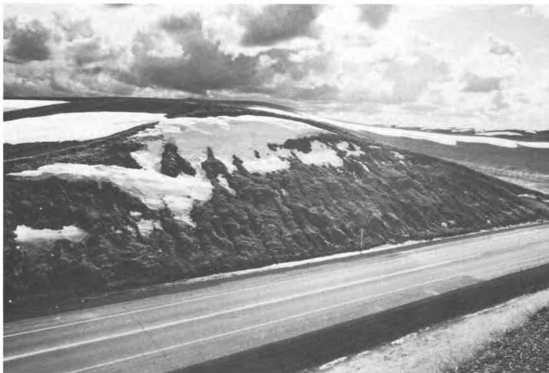
Figure 19. North-facing slope (counterpart of slope in Figure 18) exhibits slide scar and severe gully erosion.
