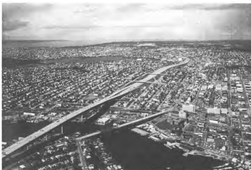
Aerial view to the north-northwest of the Interstate Highway 5 bridge over the Lake Washington Ship Canal, Seattle. Photograph by R. W. Galster, February 1971.
