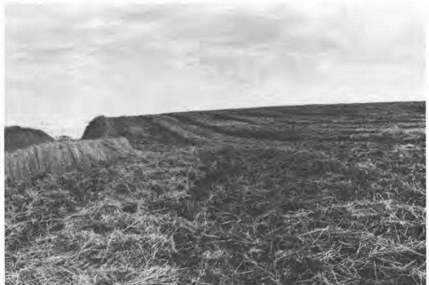
Figure 15. Low area at the center of the photograph is the runoff source causing the erosion shown in Figure 14. Cut slope is on the left.
