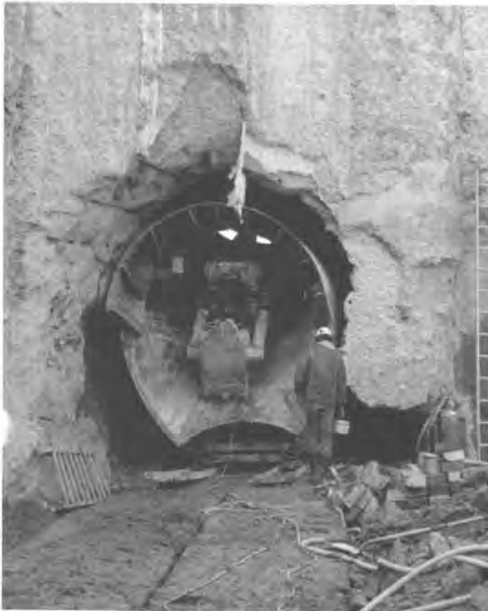
Figure 10. Breakout of drift #13 shield in east access pit.
