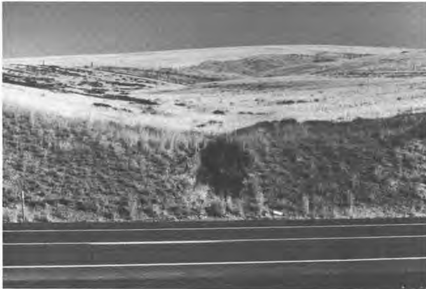
Figure 12. Erosion of loess by flow over the face of a cut (near La Crosse).
