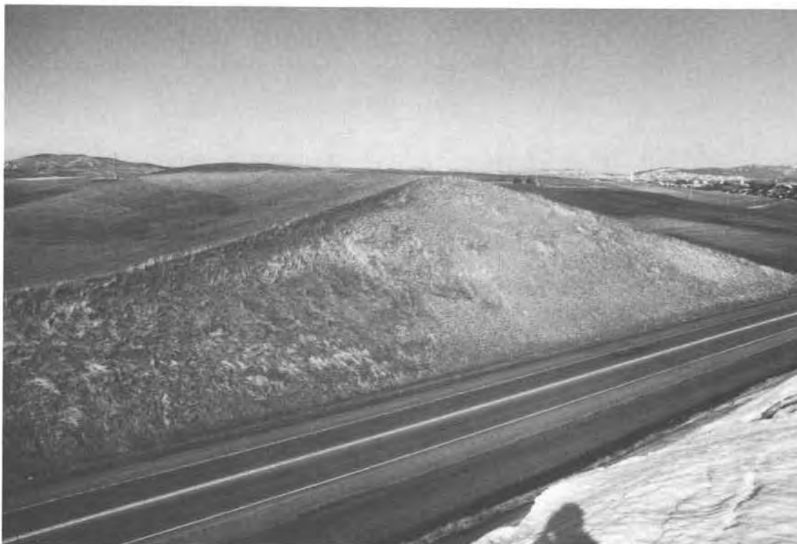
Figure 18. South-facing slope near Pullman shows little degradation. Cut is about 60 ft high.
