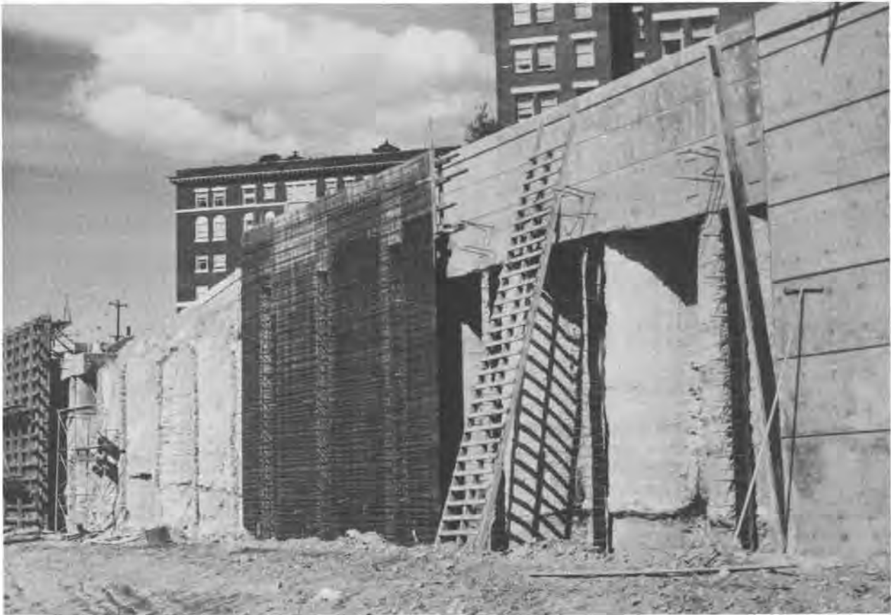
Figure 11. Cylinder piles (10-ft diameter) with permanent face walls under construction.
