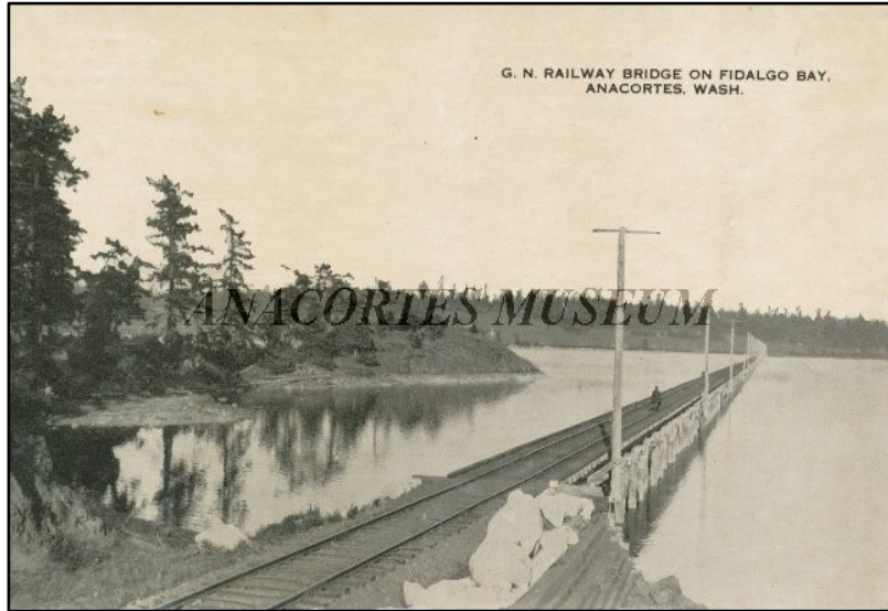
Figure 21. Photo from 1907 of Great Northern Railroad trestle looking east from Weaverling Spit. Note wooden piling construction of entire trestle prior to causeway construction. (Anacortes Museum)
